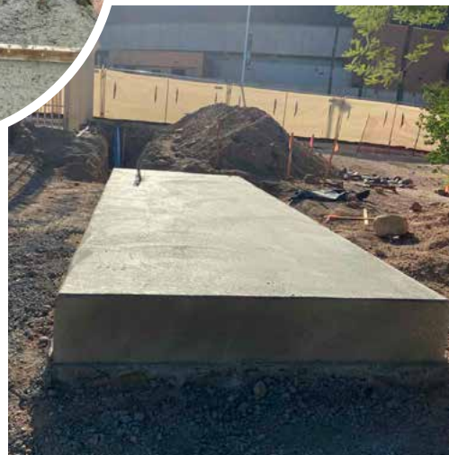
This concrete pad (pictured above) is for a generator that will serve both GCRB and Meinel West.
