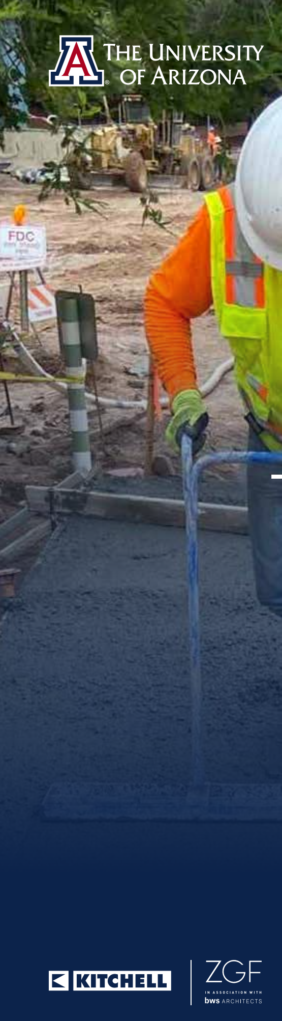
This concrete pad (pictured above) is for a generator that will serve both GCRB and Meinel West.
