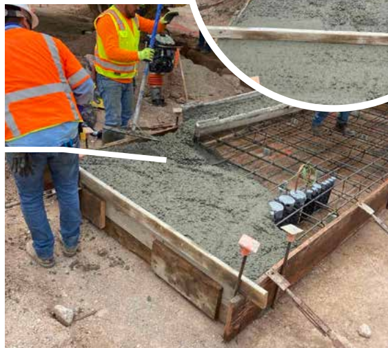
This concrete pad (pictured above) is for a generator that will serve both GCRB and Meinel West.
