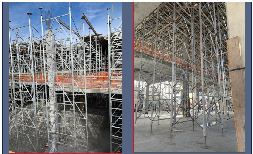
40' Towers Are Set
