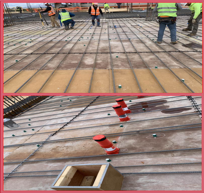
MEP Hangers and Block-outs on Level 3 Deck
