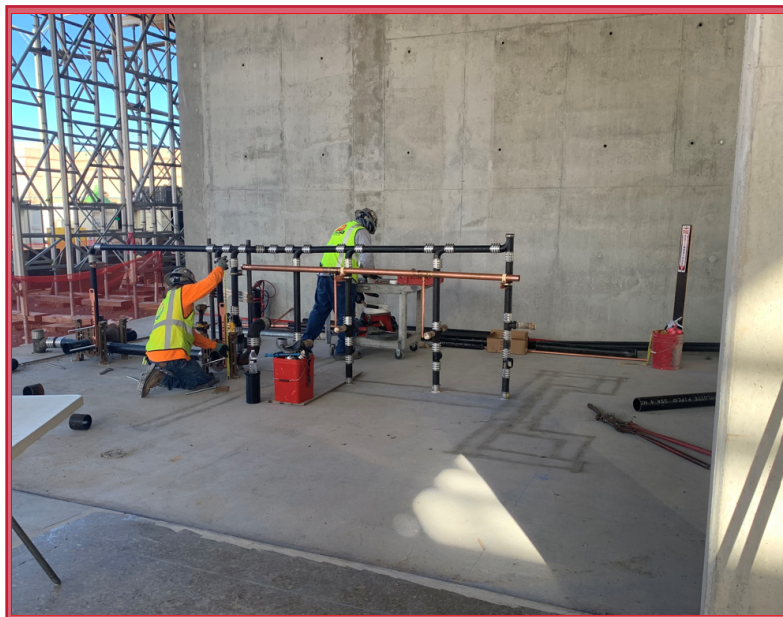
Level-1 Restroom In-wall Plumbing
