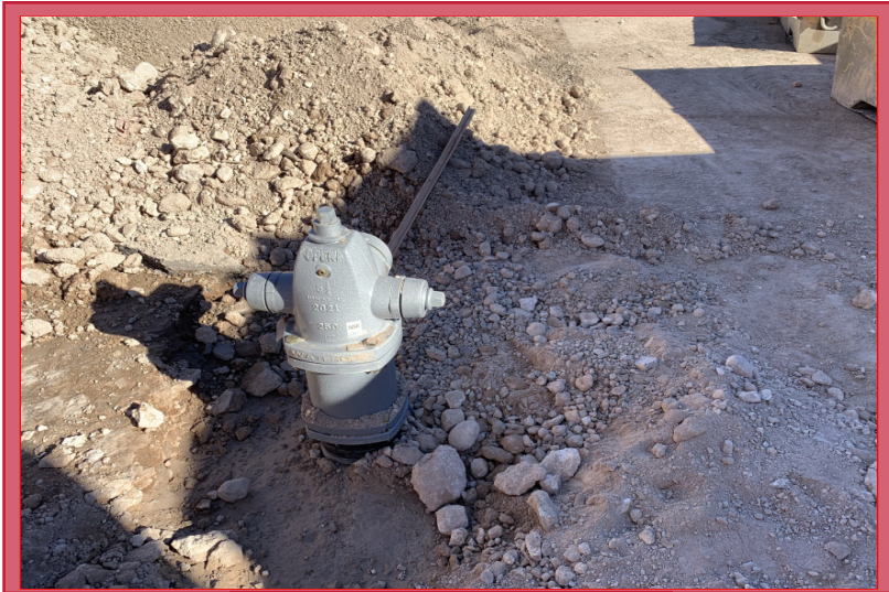
Fire Hydrant Installed on-site
