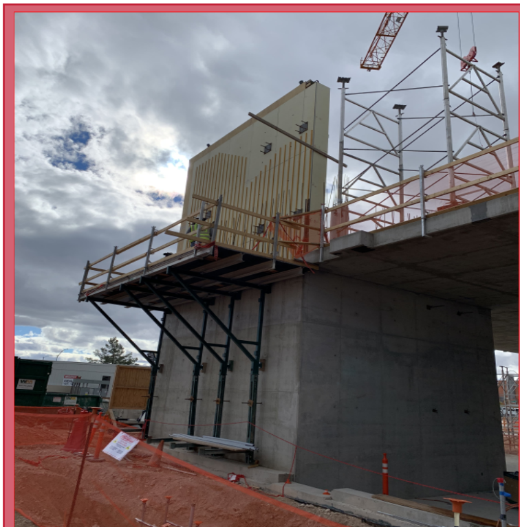
Stair-3 Level-2 Reveals Wall
