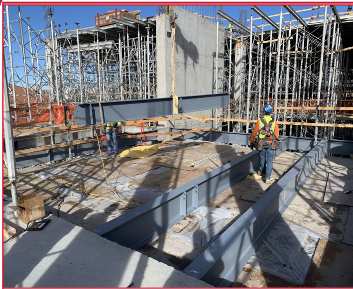
Over TV-Chamber Structural Steel Beams
