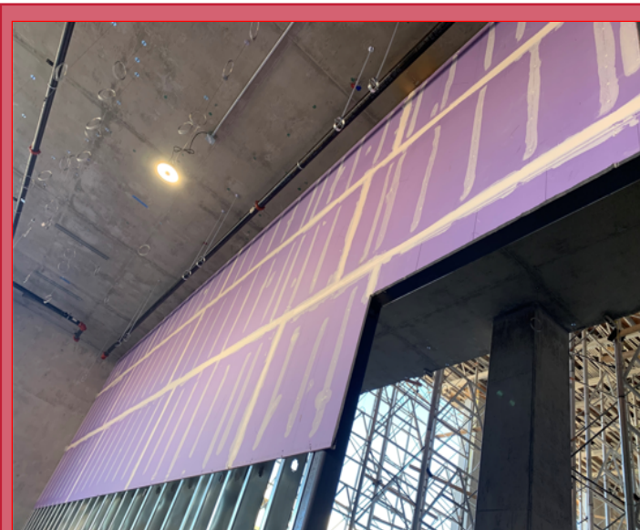
Rated Walls Tape and Prep
