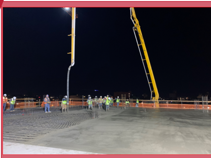
Level 3 South Slab Finishing
