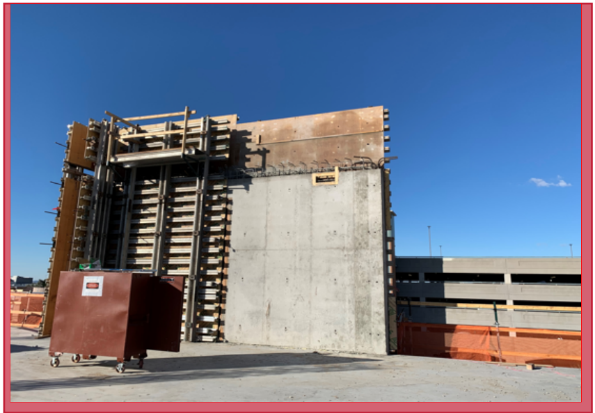
Stripping L3 Shear Wall-1
