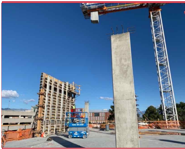
Closing L3 Shear Wall-2
