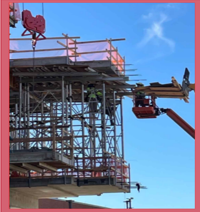
Stripping Level 3 Deck
