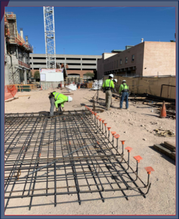
Pre-Fabricating Level 3 Walls
