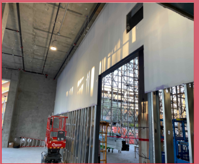
Dry Wall Started - West Corridor
