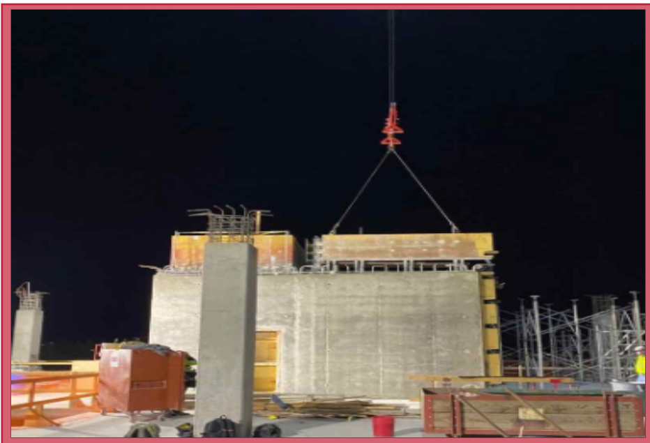
Stripping Core Wall-1
