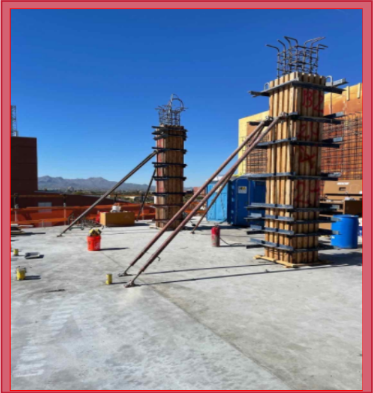
Setting Level 3 Columns
