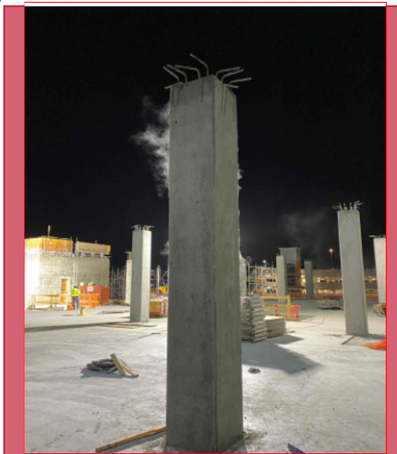
Stripping Level 3 Columns
