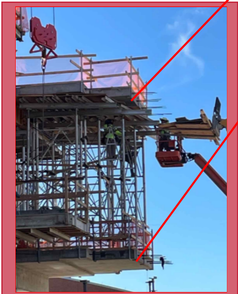
Northwest Building Cantilever Current Progress
