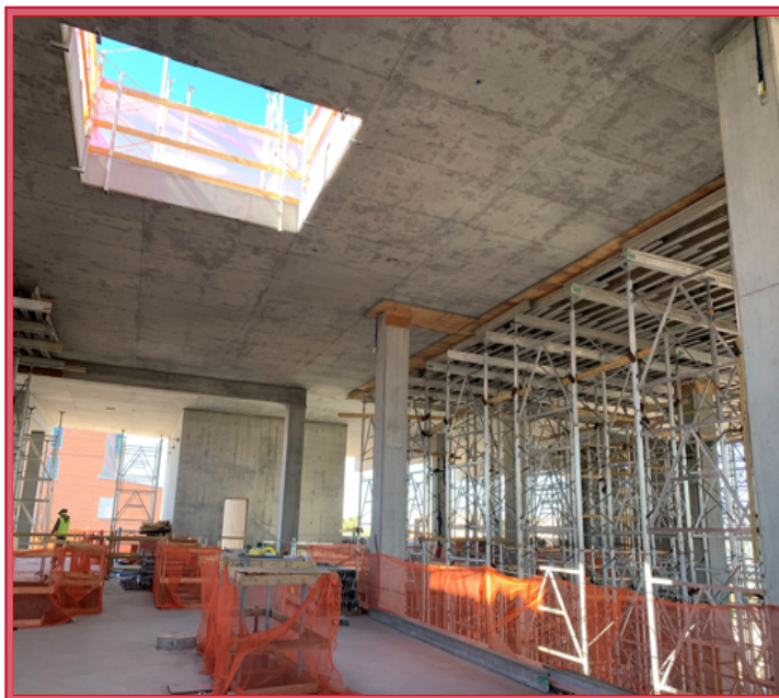
Stripping Level 3 Deck
