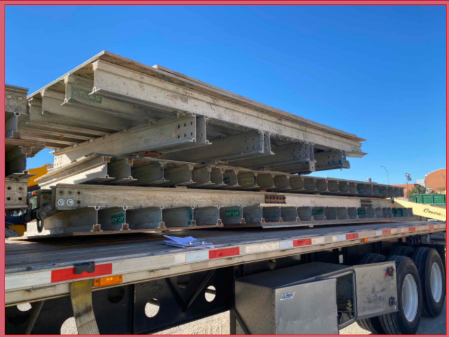
Demobilizing Vertical Form Work
