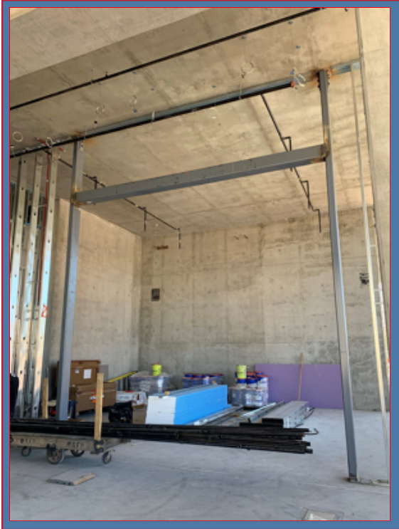
Shaker Room Coiling Door Steel
