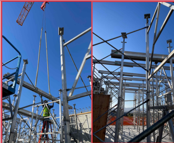
Setting Level 4 Deck Stringers
