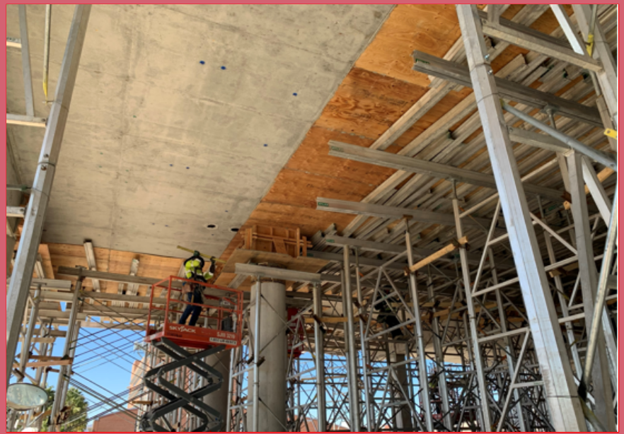
Stripping Level 3 Deck
