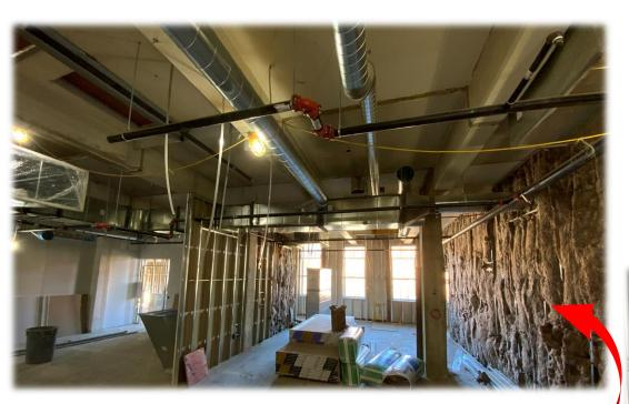
**Level 2:** Overhead HVAC is in; Fire protection piping is in, and walls are starting to be insulated and closed-up.
