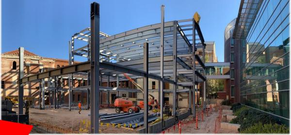
Structural steel is complete on the east side of the new building - "The Commons". Stay tuned for the west side to be complete and steel deck to be set in place.
