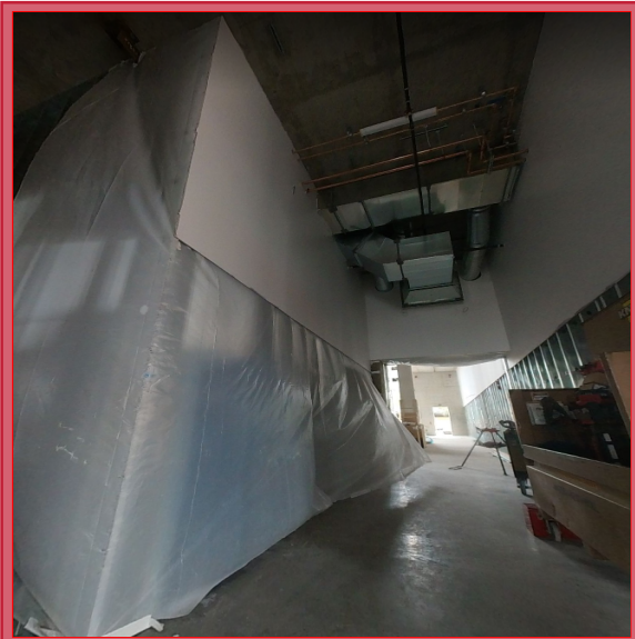
Level-1 Wall Vapor Barrier
