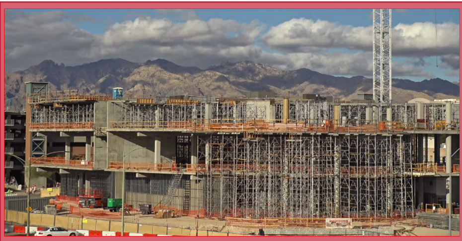
Facing North View
