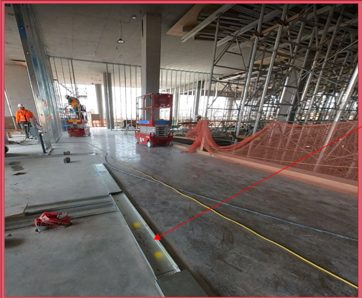
Level-2 Framing Track
