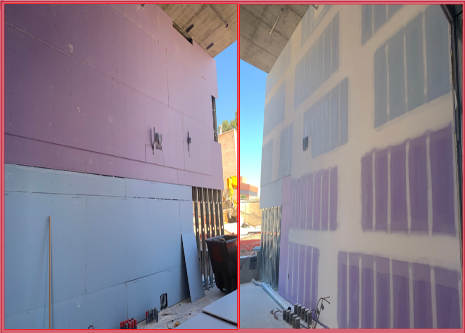
Level-1 Electrical Room Sheeted and taped
