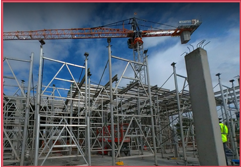
Level 4 South Slab Decking
