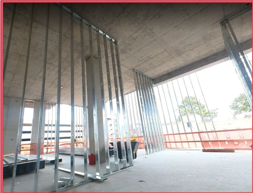
Level-2 Interior Walls Framing
