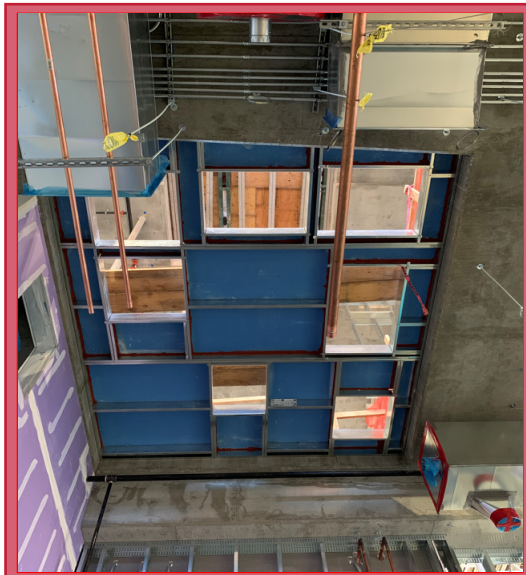
West Mechanical Shaft
