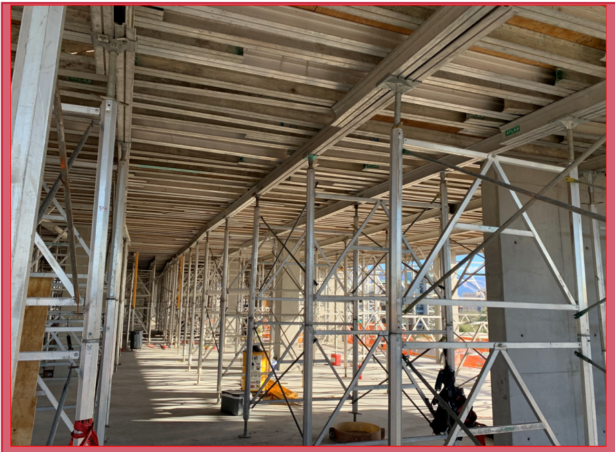
Level-4 Deck Shoring Towers
