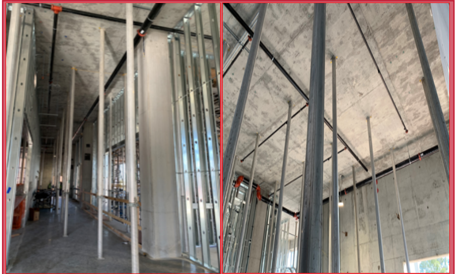
Re-shoring Post for Level-4 Deck On Level-2
