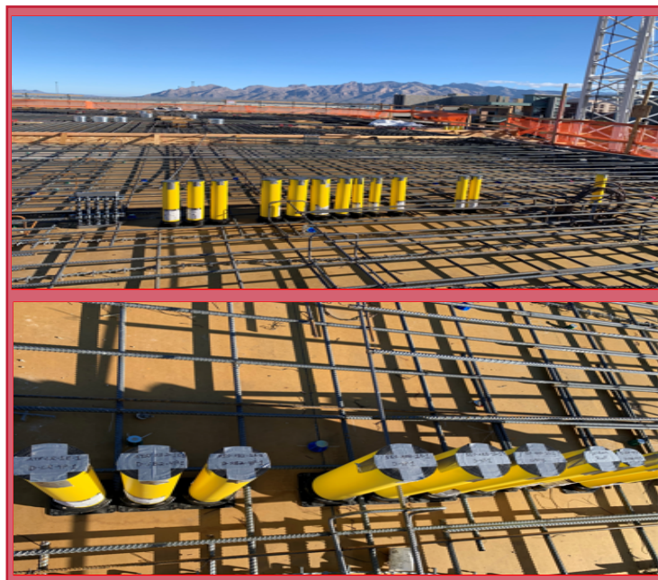
Level-4 MEP Blockout
