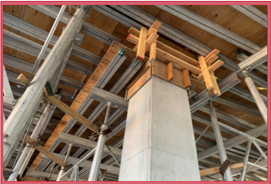
Level-4 Beam Form-Work
