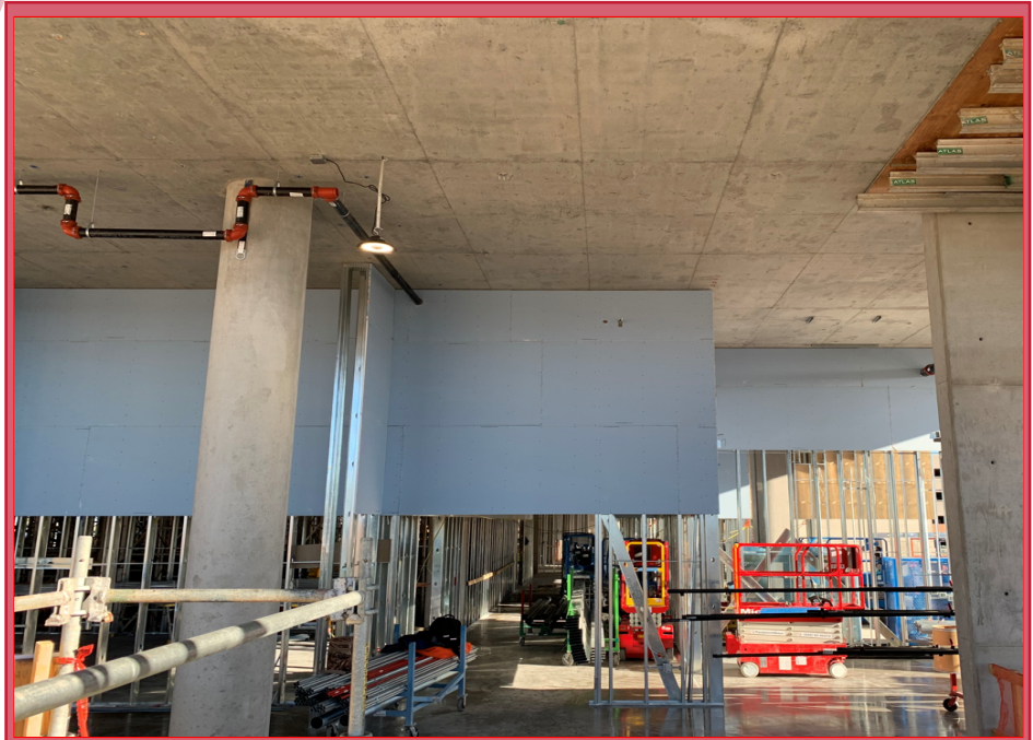
Level-2 Topping-Out Drywall
