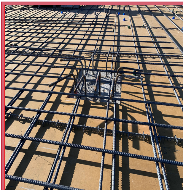
Level 4 Deck (Roof) Reinforcing
