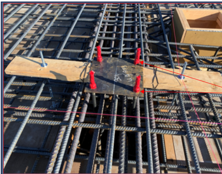
Mechanical Room Steel Structure Anchor Bolt
