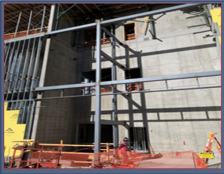
East Elevator Steel South Connection
