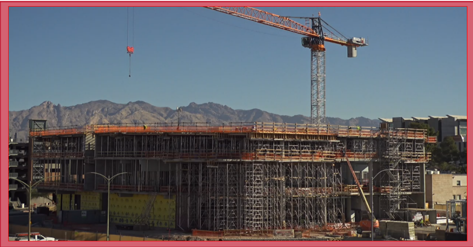
Facing North View
