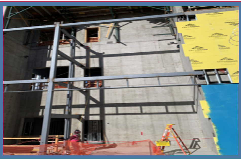
East Elevator Steel North Connection
