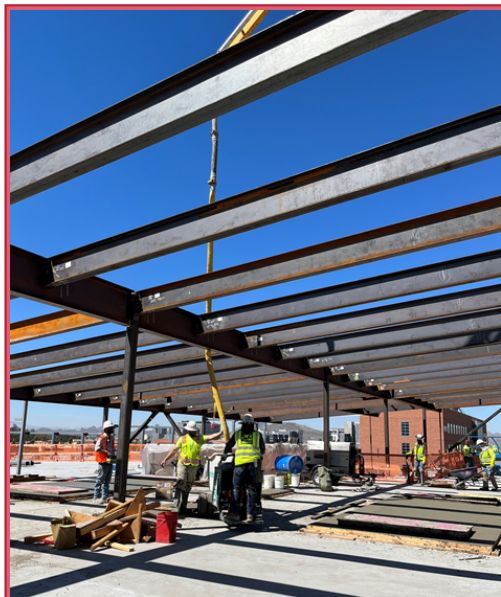
Level 4 - Pouring Equipment Pads
