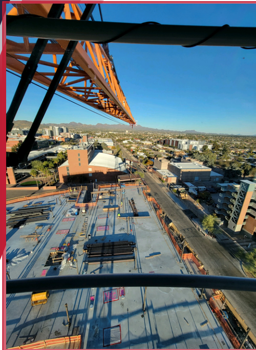
View from Crane
