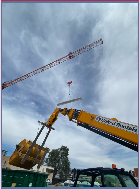
Topping Out Beam Dry-fitting
