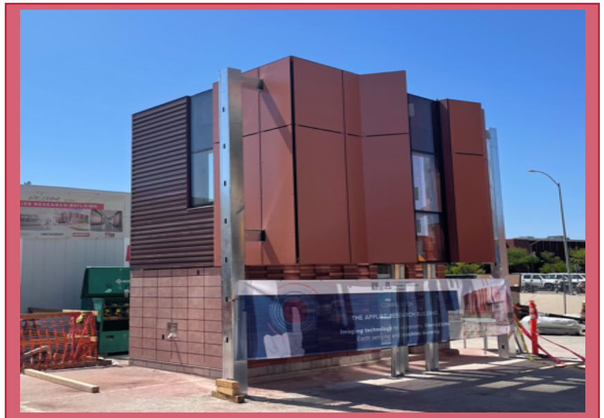
Exterior Elevation of Mock-Up
