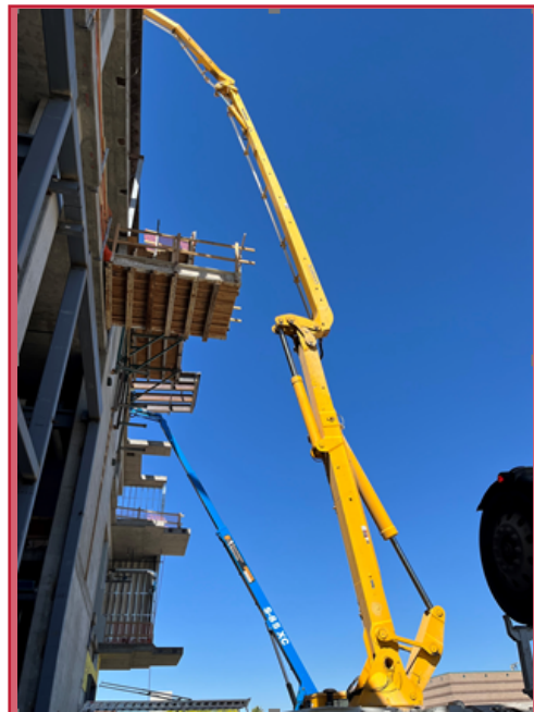
Concrete Pump Truck
