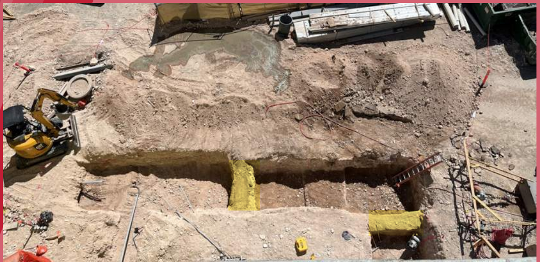
Aerial View of East Yard Excavation
