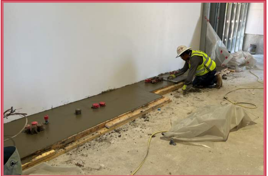
Finishing of L1 Concrete Equipment Pad
