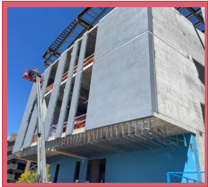
Masonry (Blue) Waterproofing on L1
