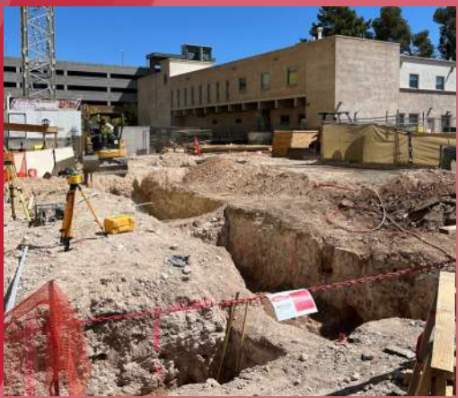
East Yard Excavation
