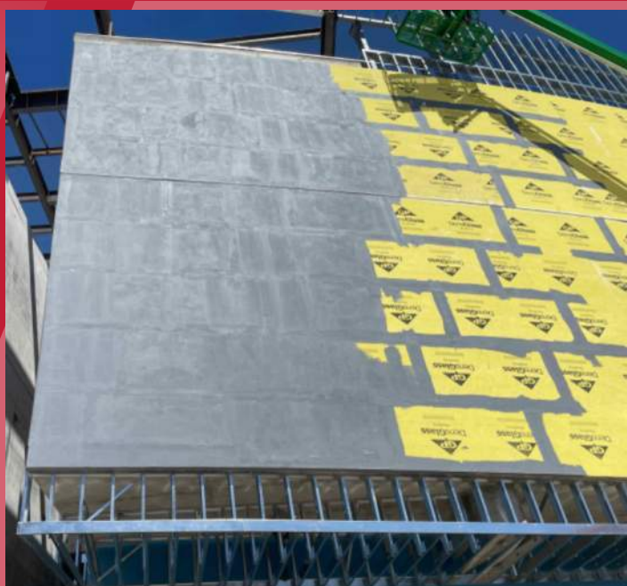
Metal Panel Facade (Gray) Waterproofing L2-3
