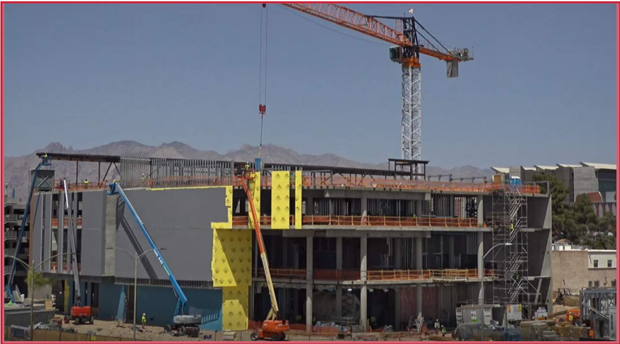
North Elevation View
