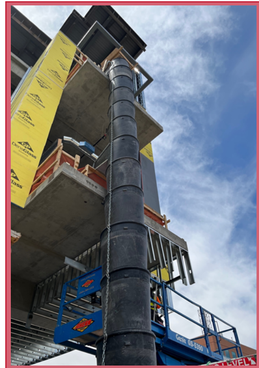
North Elevation Trash Chute
