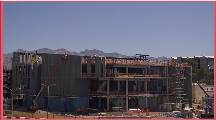
North Elevation View
