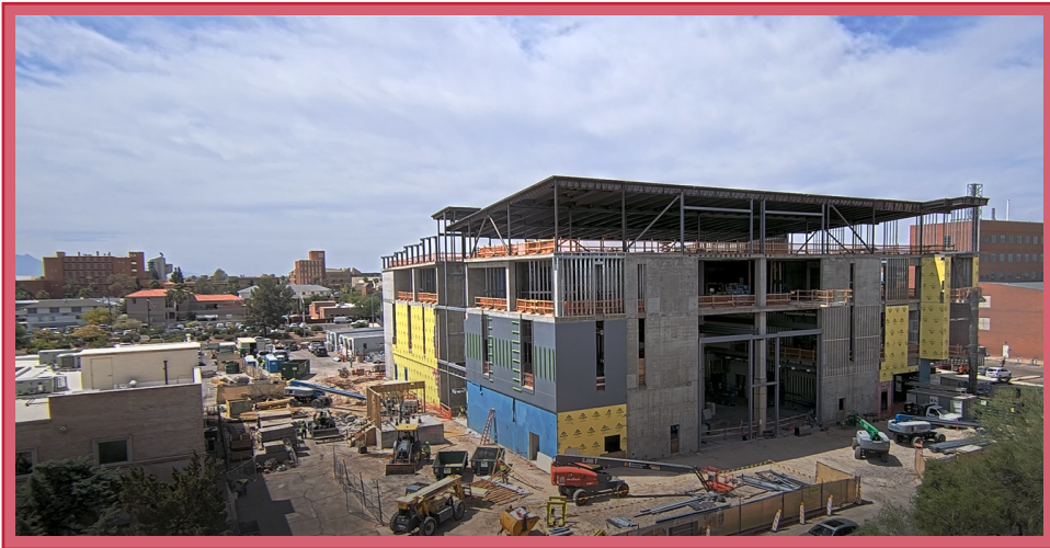
South Elevation View
