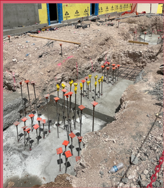
East Yard Reinforcing
