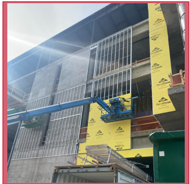
North Exterior Elevation Framing
