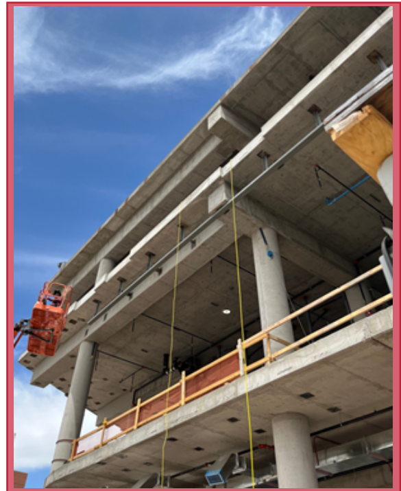
Level 3 Soffit Steel for Exterior Glazing
