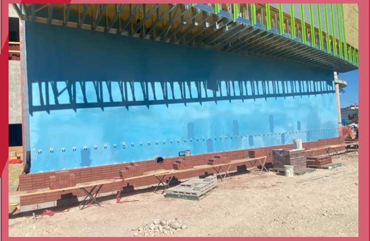
West Elevation Masonry
