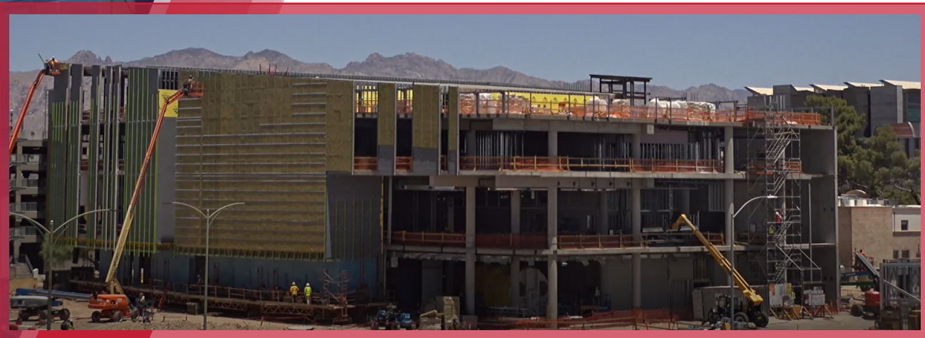
Facing North View
