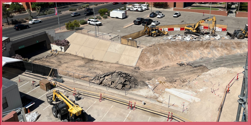
Construction is underway
