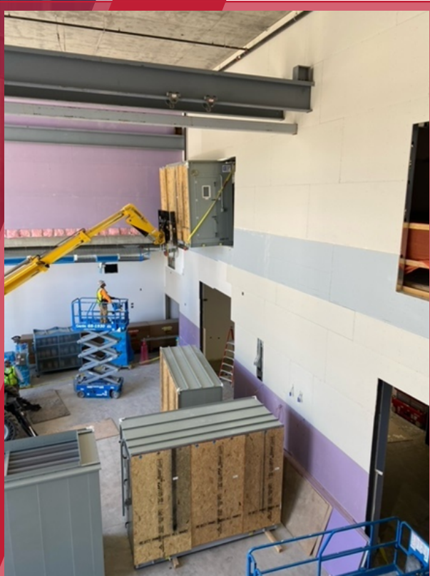
Air Handler forklifted to Level 2
