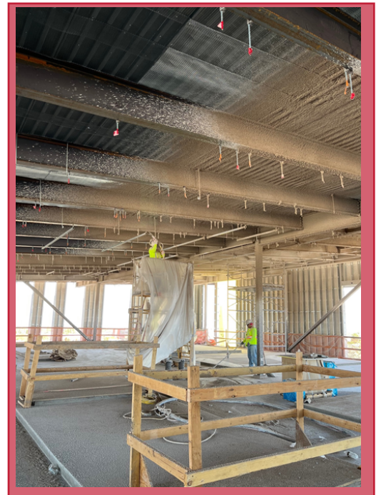
Spraying Cementitious Fireproofing
