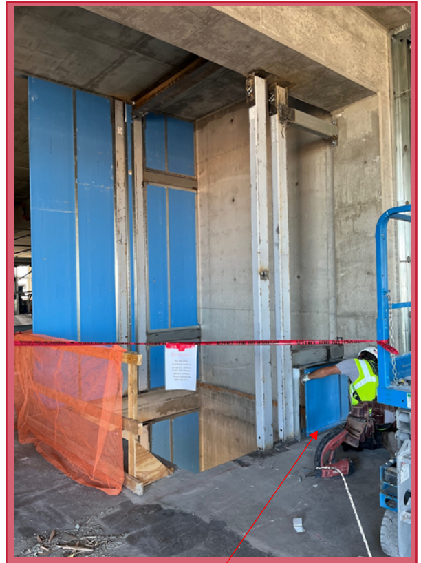
Framer installing 2-hour fire rated wall
