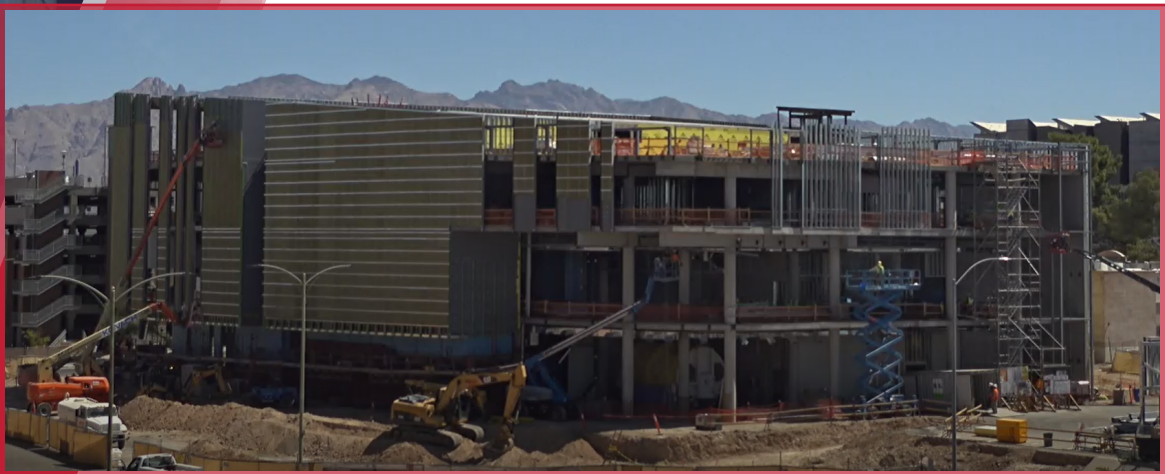
Facing North View
