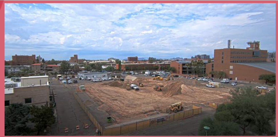
View Looking South Toward Speedway from Helen Street - Building Pad Prep
