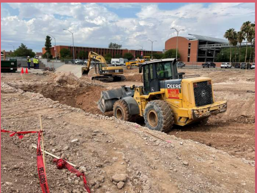
Elevator Pit Excavation
