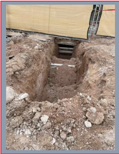
Chilled water piping trenching and installation
