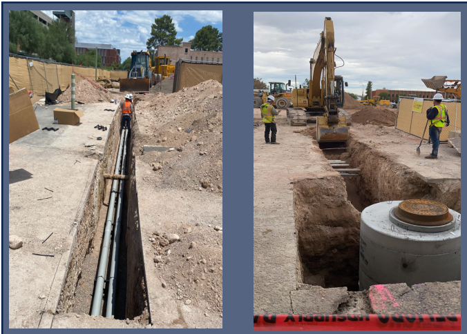
Helen Street Communications and Sewer Installation
