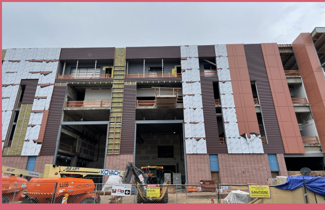
North side in progress
