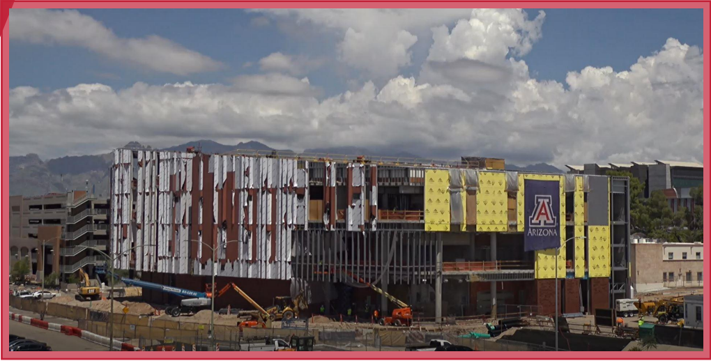
Facing North View
