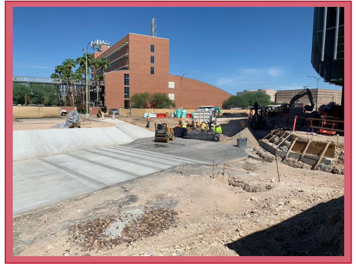
Crews Setting Asphalt with Paving Machine
