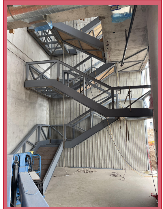
Stair #3 at SE Corner Guardrail
