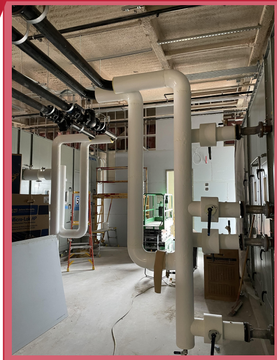
Level 4 Air Handler Units Mechanical Fit-out Progress
