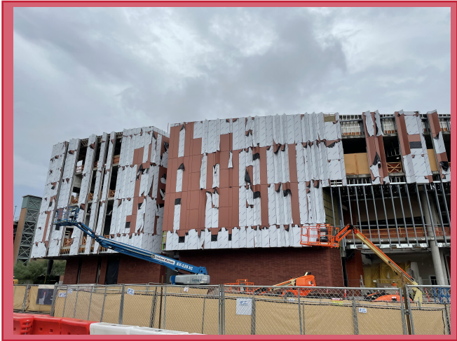
West side exterior in progress
