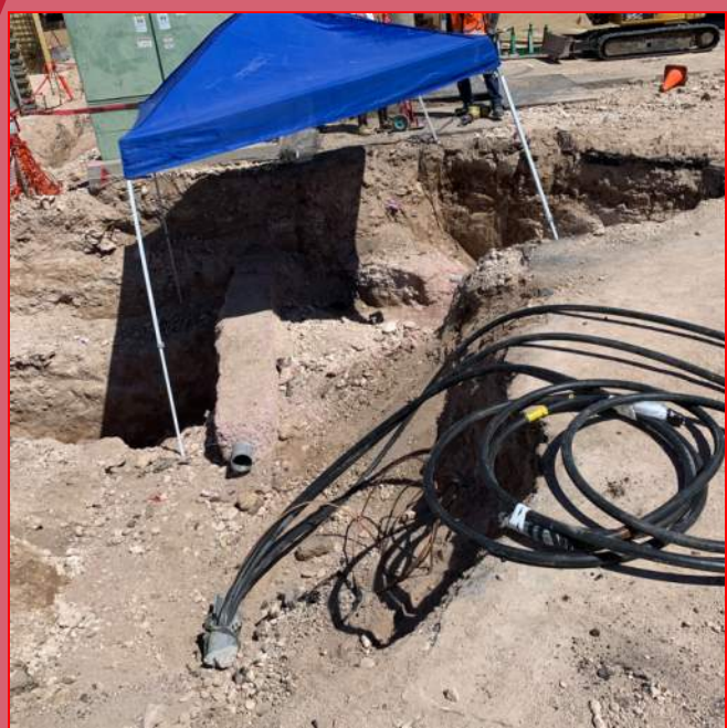
South-Loop In Progress
