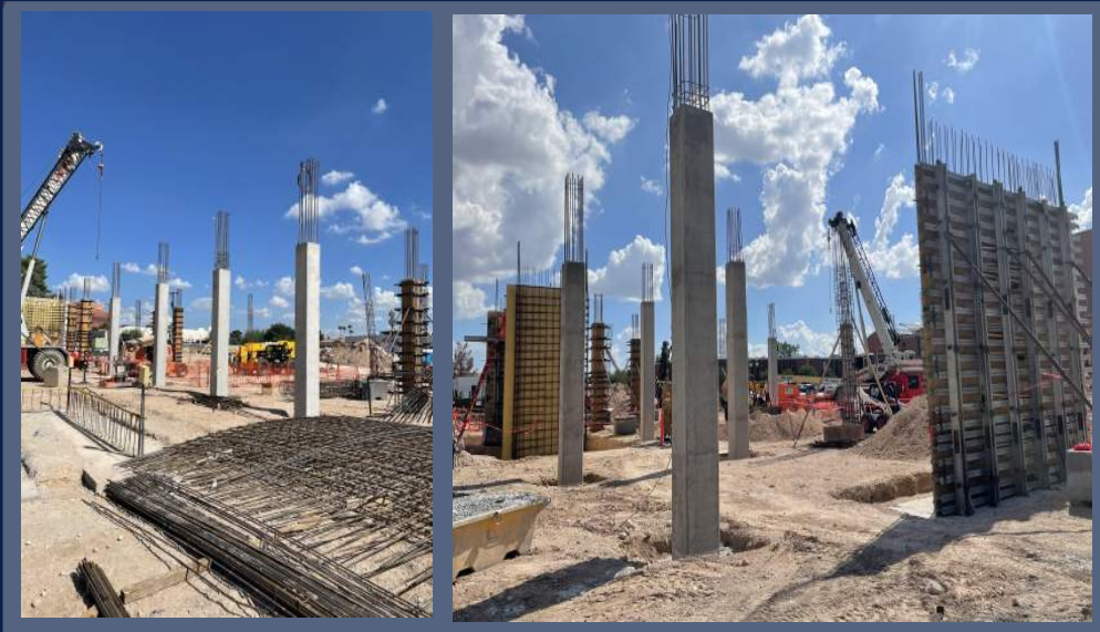
Column Stripped and Walls Formed
