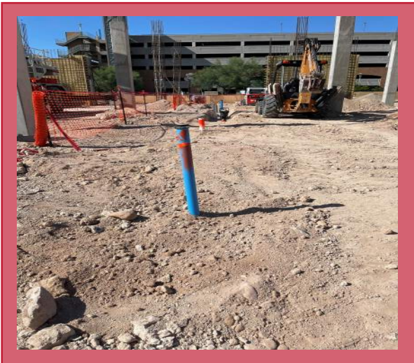
Lab Waste and Main Waste Lines Complete and Inspected
