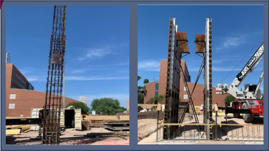
Embeds Installed and Core 2 Formwork
