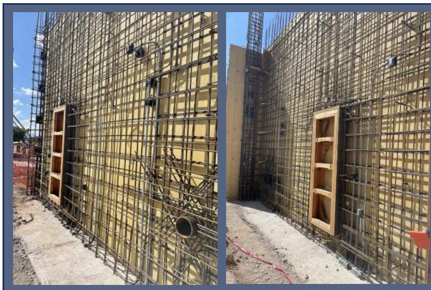
In Wall Electrical Rough-in
