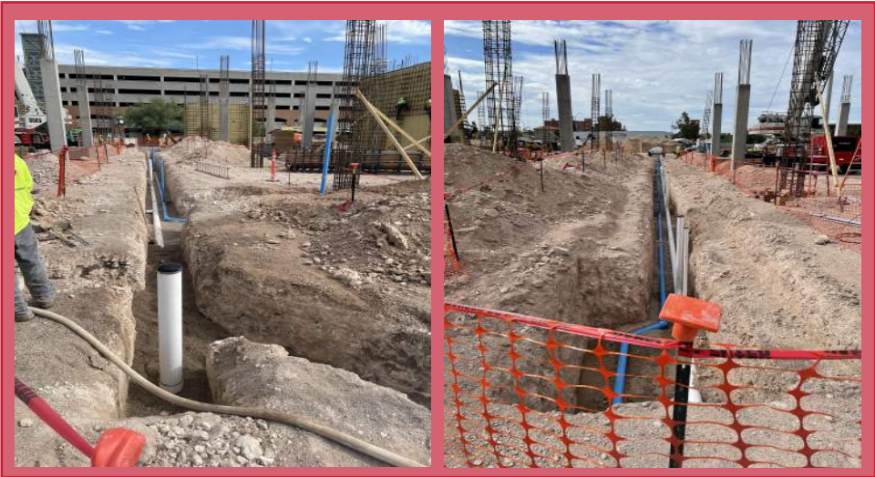
Lab Waste and Main Waste Lines Complete and Inspected
