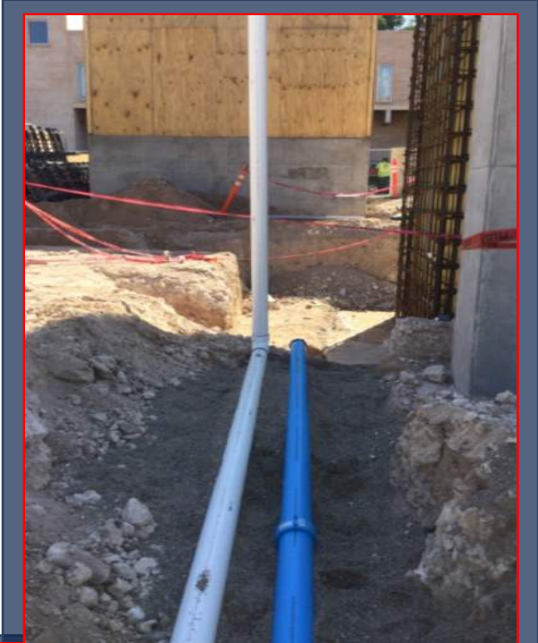
Site Waste and Sanitary Line Branches
