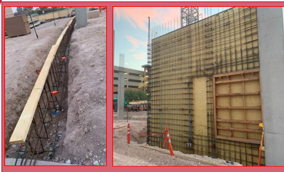
Building Continuous Footing and Shearwall-3 Reinforcing
