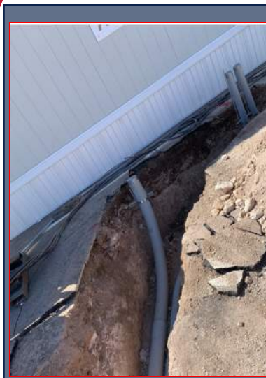
Site Permanent Power Connection
