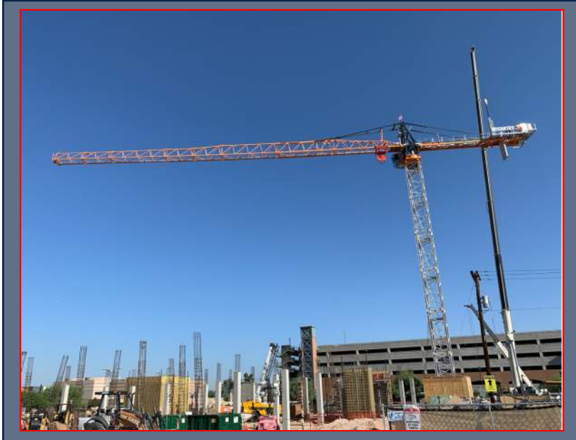
Tower Crane Assembly Completed
