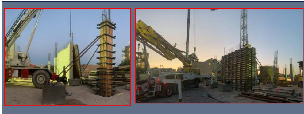
Shearwall-1 Stripped and Shearwall-2 Poured
