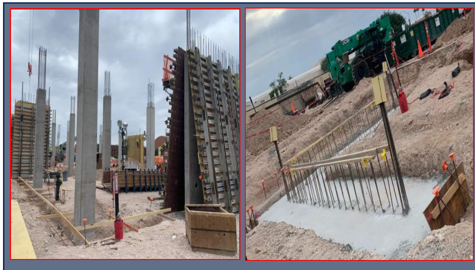
Shearwall 2 Stripped & Last Grade Beam Poured
