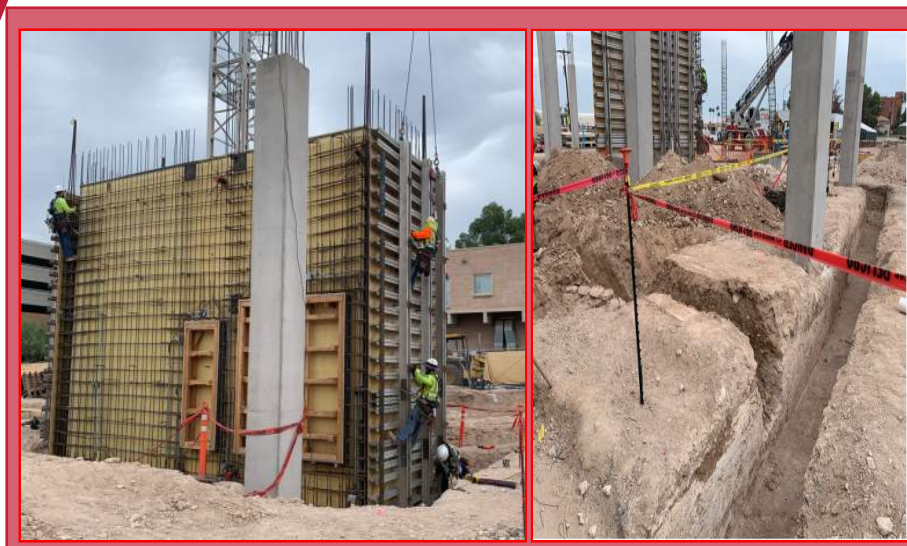
Core Wall-2 Being Closed & Continuous Footing Clean Cut
