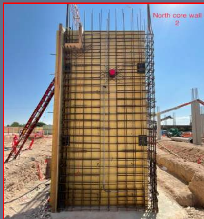
Core Walls Reinforcing
