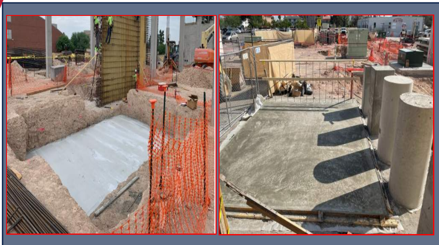
Thermal Vacuum Pad Base & Slab On Grade Mock-up
