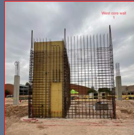
Core Walls Reinforcing
