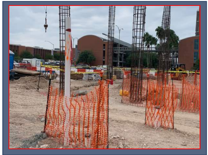
Sanitary Line Branches Stub-ups
