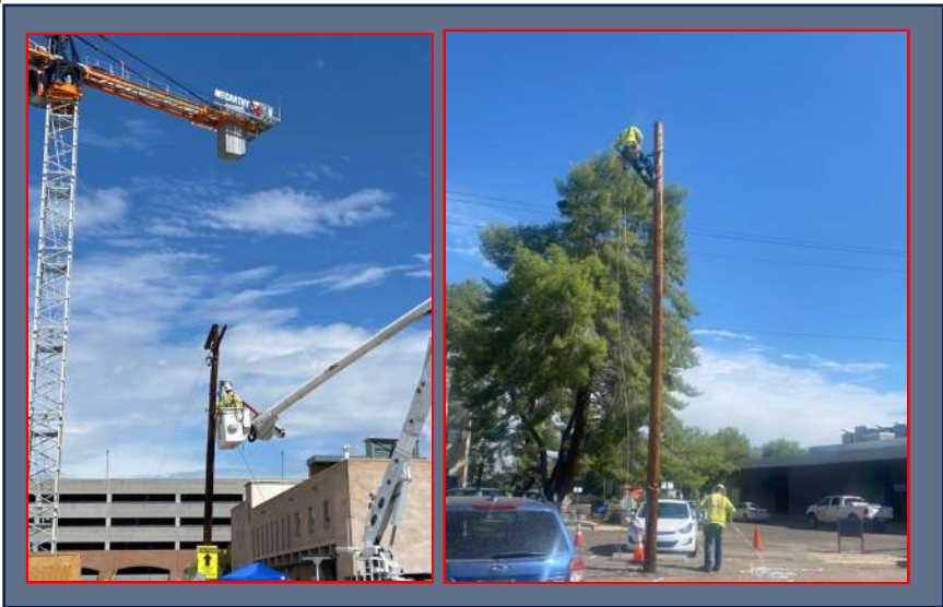
TEP Pole Removal
