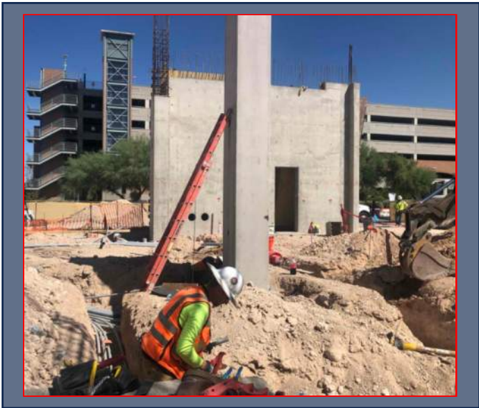
Area-1 Underground Utilities Completion
