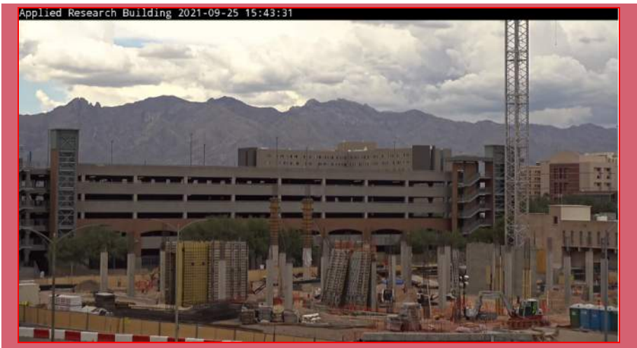
Facing North View
