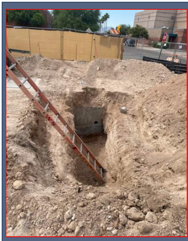
Domestic Water Tie-in From UA Tunnel
