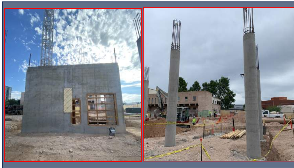
Core-2 and Round Columns Stripped
