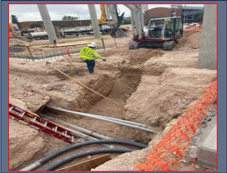
Generator/ Feeders Excavation
