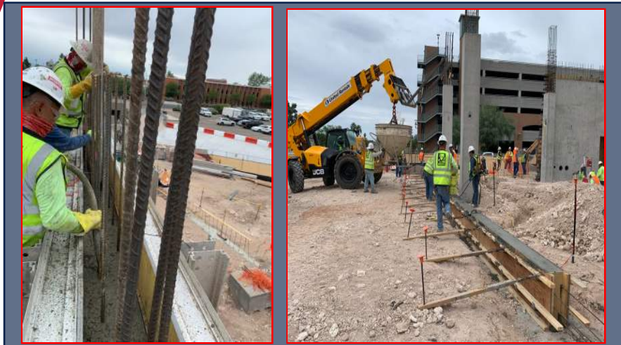
Shear Wall-3 & Stem Wall Poured
