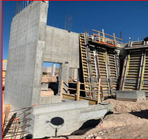
Elevator 2 Pit Wall Stripped & Dynamic Embeds Poured
