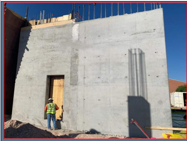
Core Wall 1 Stripped
