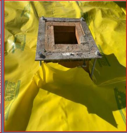
Elevator 2 Pit Wall Stripped & Dynamic Embeds Poured
