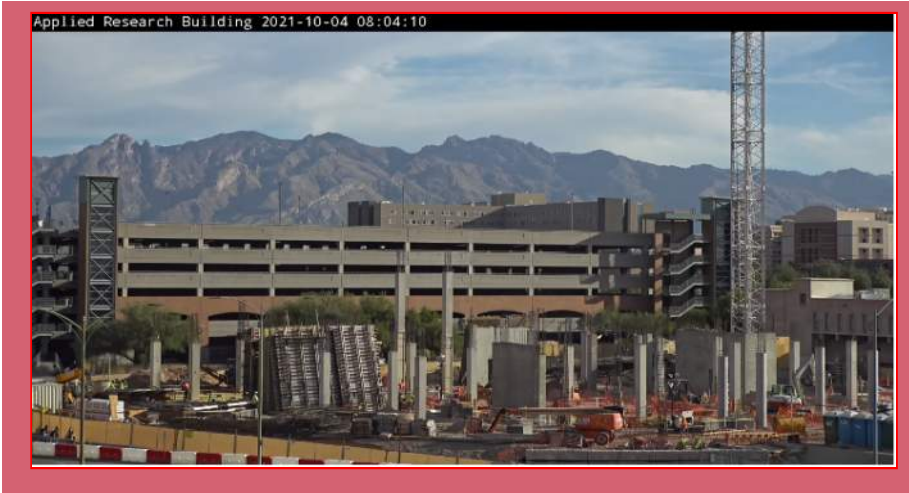
Facing North View
