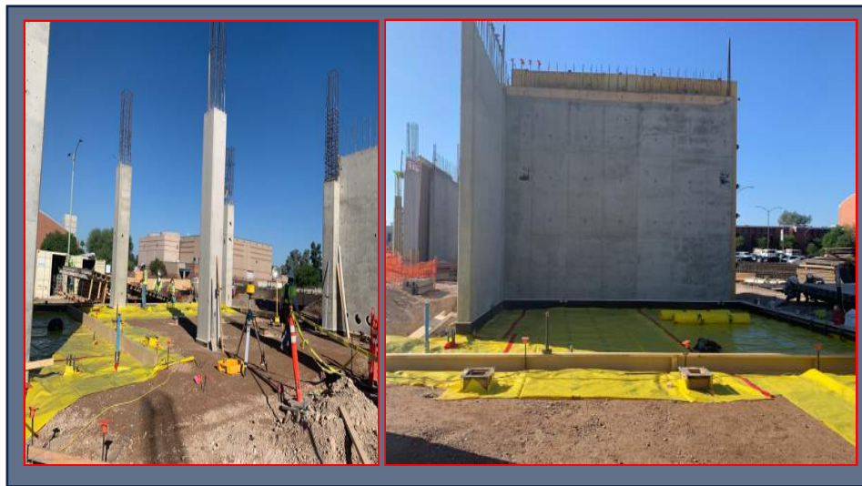
SOG Area 1 - Aggregate Base and Vapor Barrier
