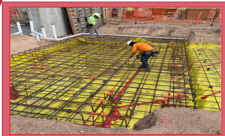
Thermal Vacuum Pad Reinforcing
