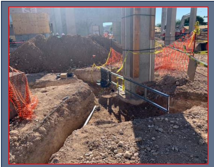
Area-2 Underground Utilities
