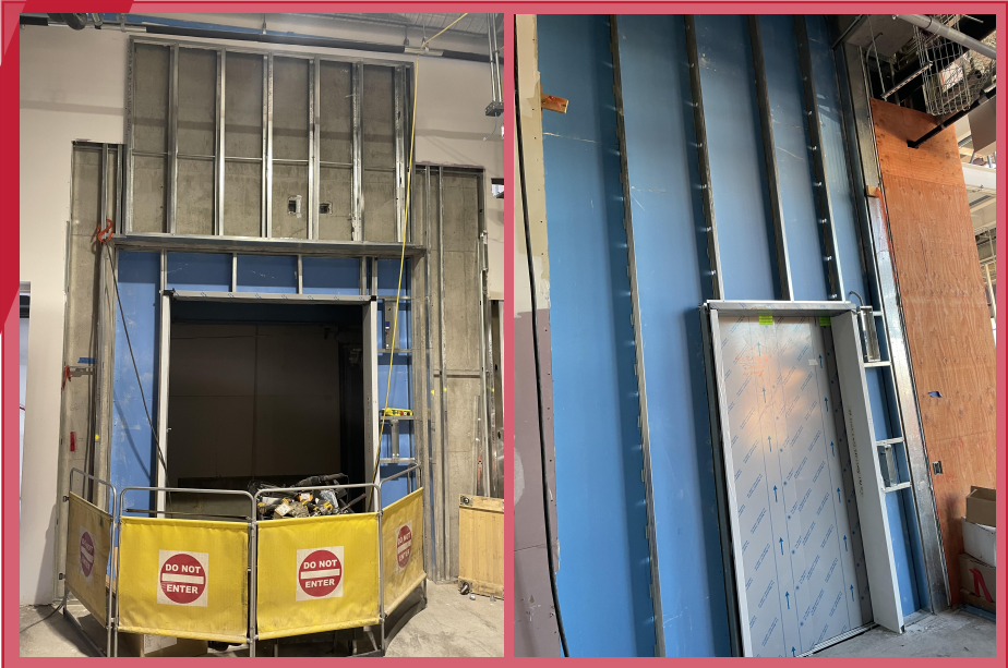
Elevator fronts for East and West elevator on level 1
