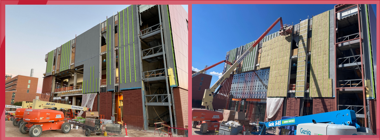
Installing green girls and insulation
