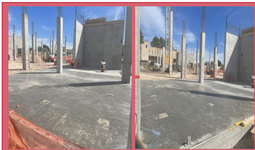
First Slab Cured
