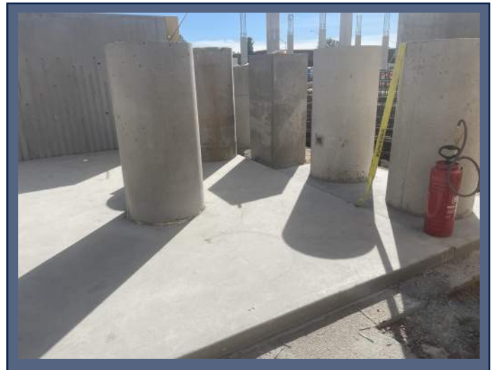
Mock-up of Level 2 Columns
