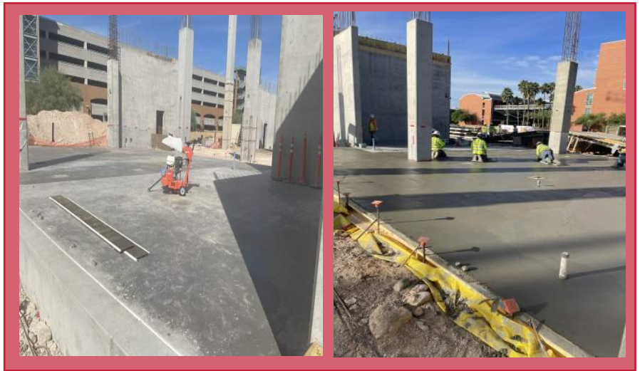
First Slab Poured
