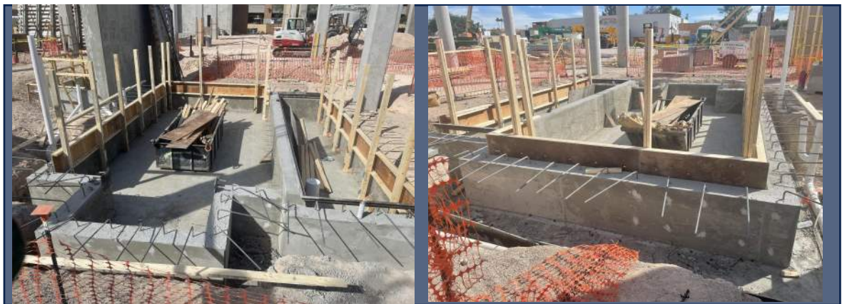
TV Chamber walls poured and stripped
