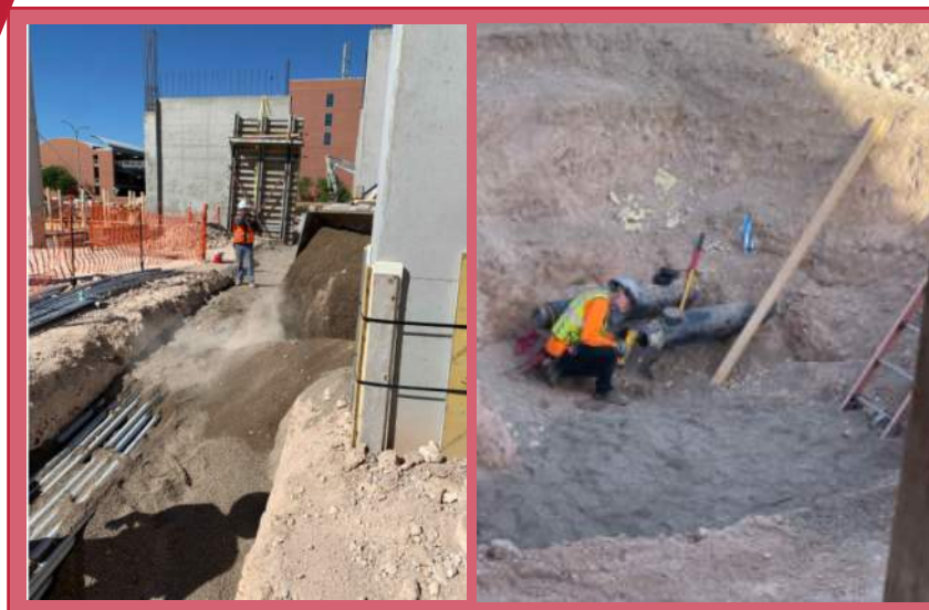
Underground Utilities Backfill & Chilled Water Line
