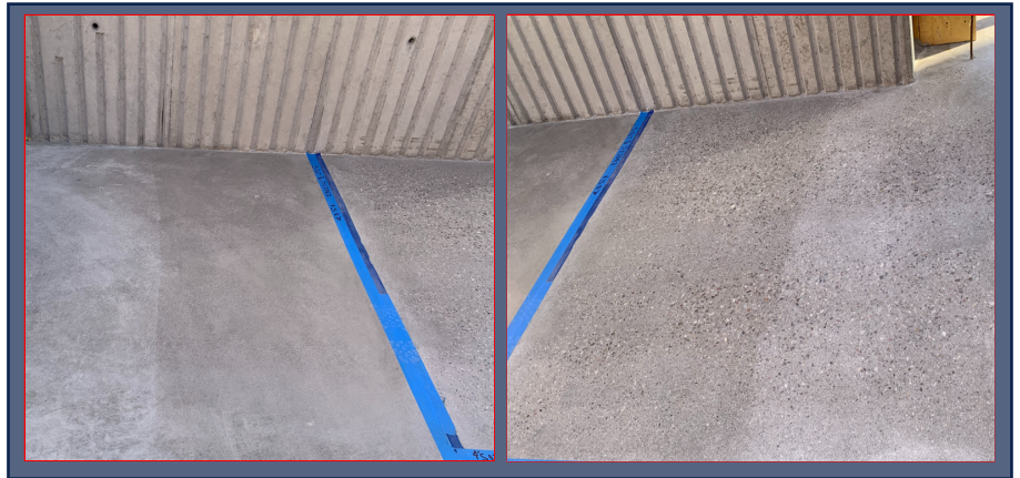
Slab on Grade Salt&Pepper and Medium Grind
