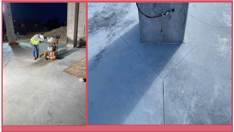
Saw Cutting NW Slab
