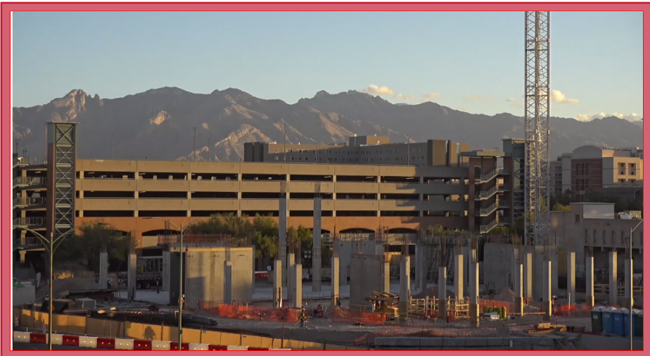
Facing North View
