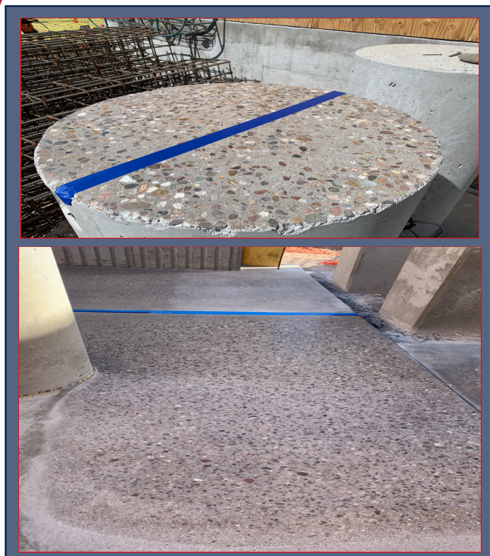
Upper Levels (Large Agg) and SOG Heavy Grind
