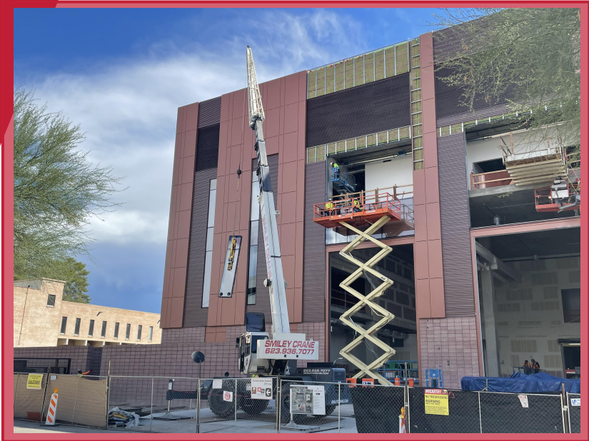
Flying a panel of glass for the North face
