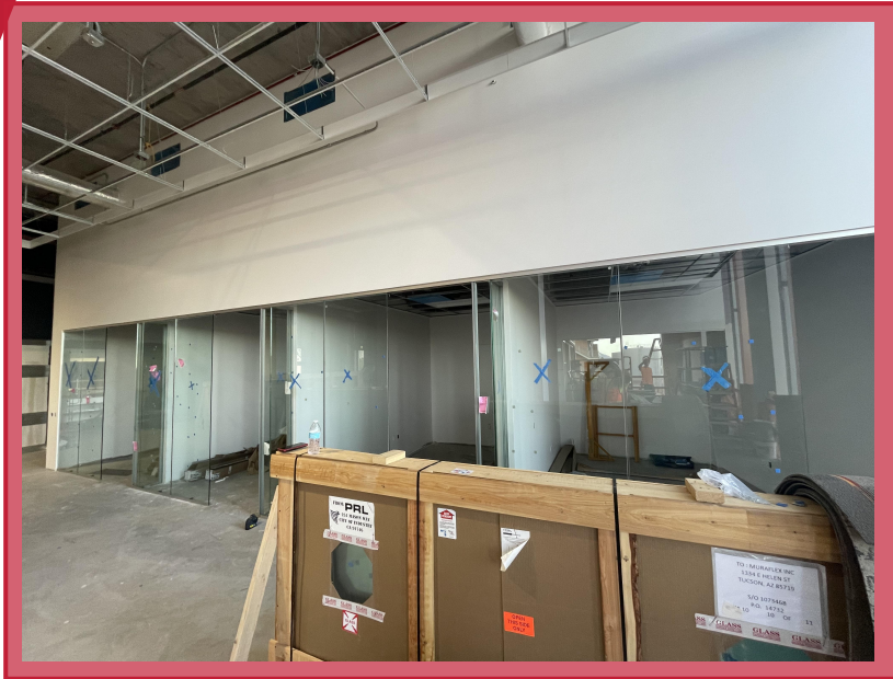
Interior glass installed for conference rooms on level 2
