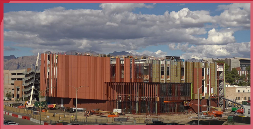
Facing North View
