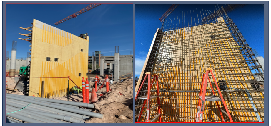
Core Wall 3 Build-up With Reveals
