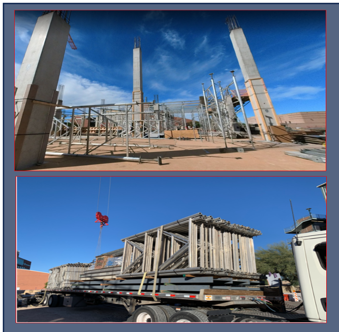
Level 2 Deck Shoring
