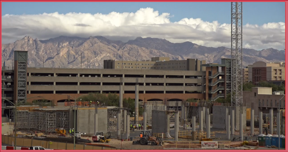
Facing North View
