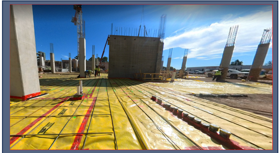
South Side of Level 1 Vapor Barrier and Reinforcing
