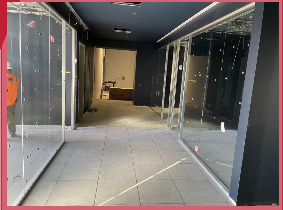
Interior glass installed on level 2
