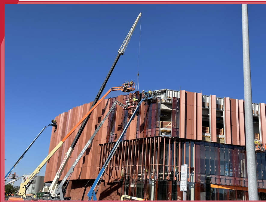
Flying a panel of glass on the West face
