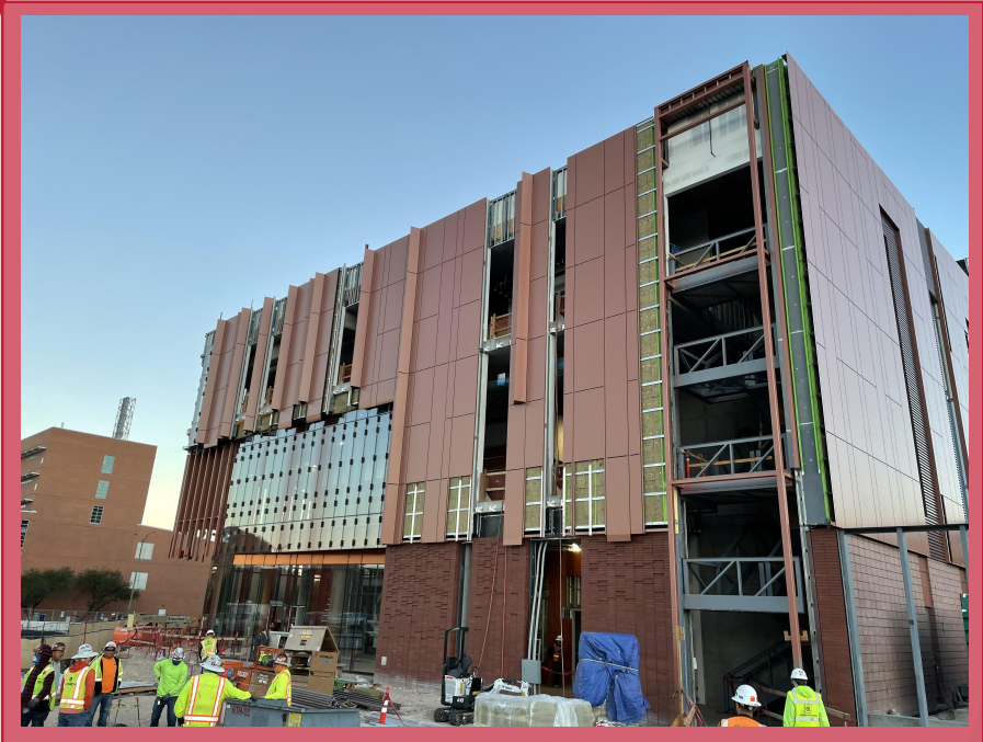
Metal panel progress on South elevation
