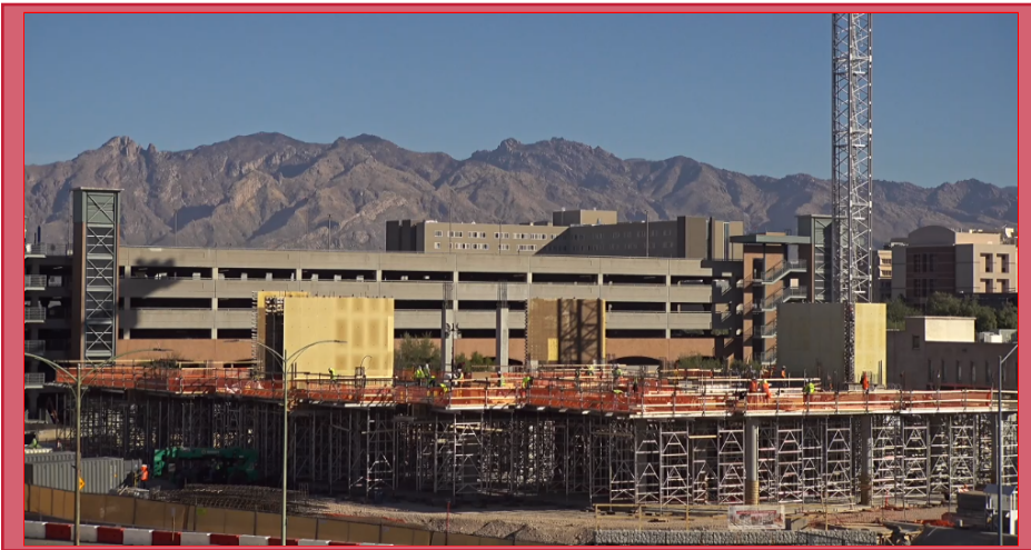
Facing North View
