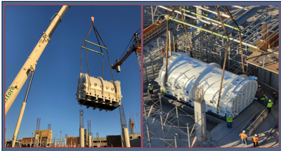
Hoisting Thermal Vacuum Chamber
