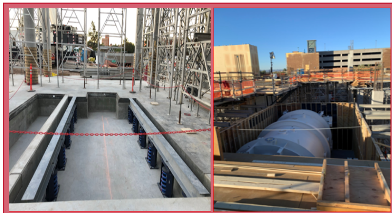
Vibration Isolation and Temporary Protection for the TV Chamber
