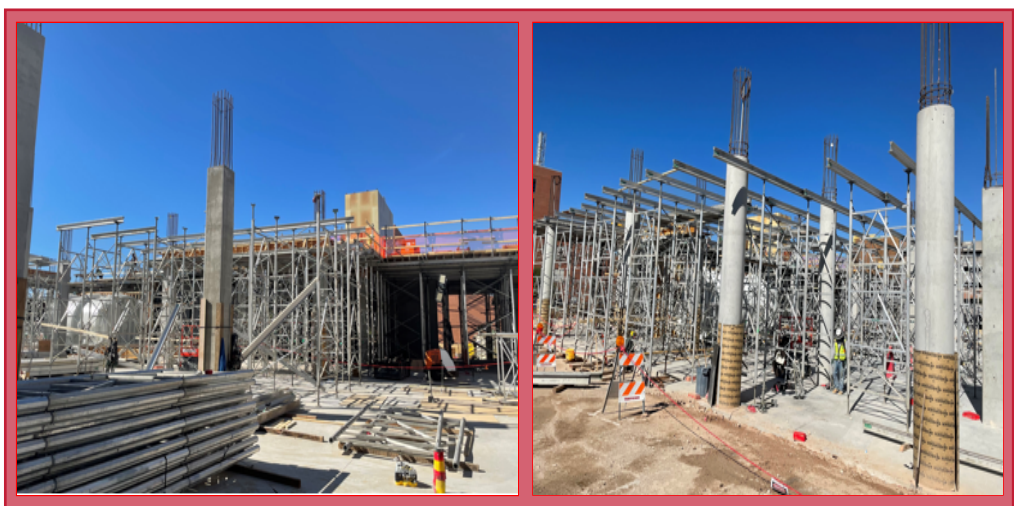
Level 2 Deck Shoring
