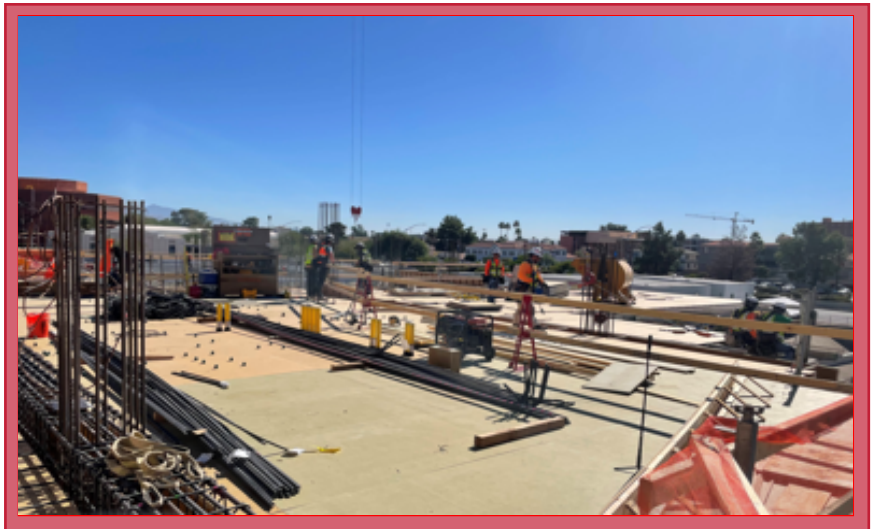
Level 2 Deck Sheeting
