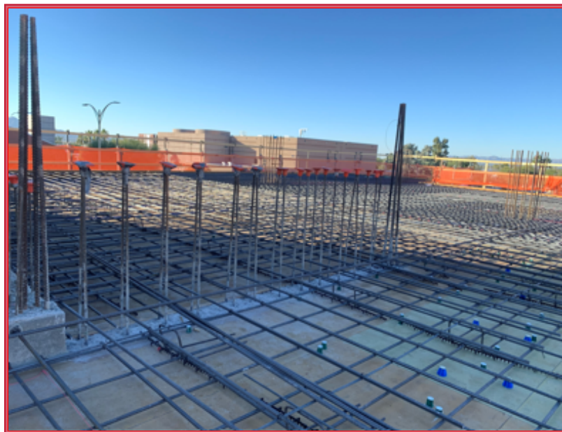
Level 2 Deck Top Mat Of Reinforcing
