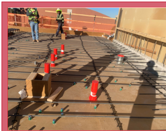
Mechanical and Plumbing Rough Blockouts and Sleeves
