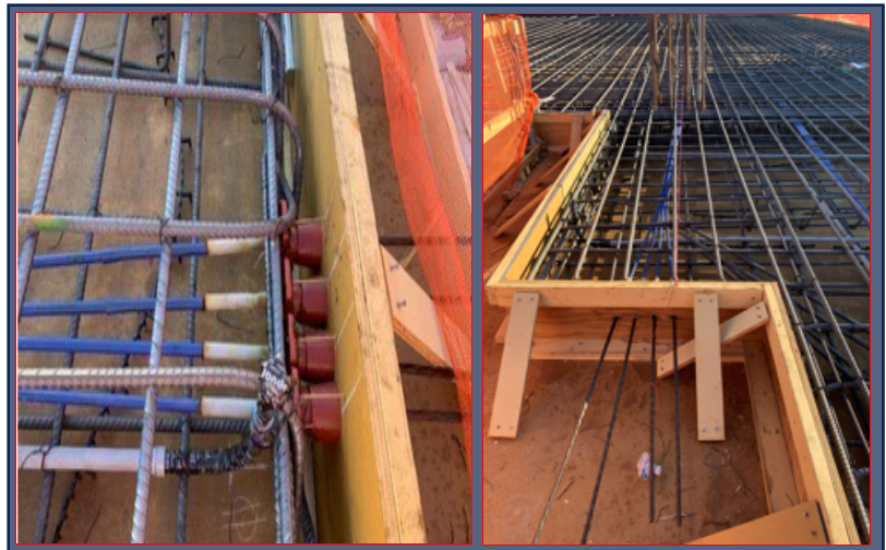
Post Tension Cables Installed
