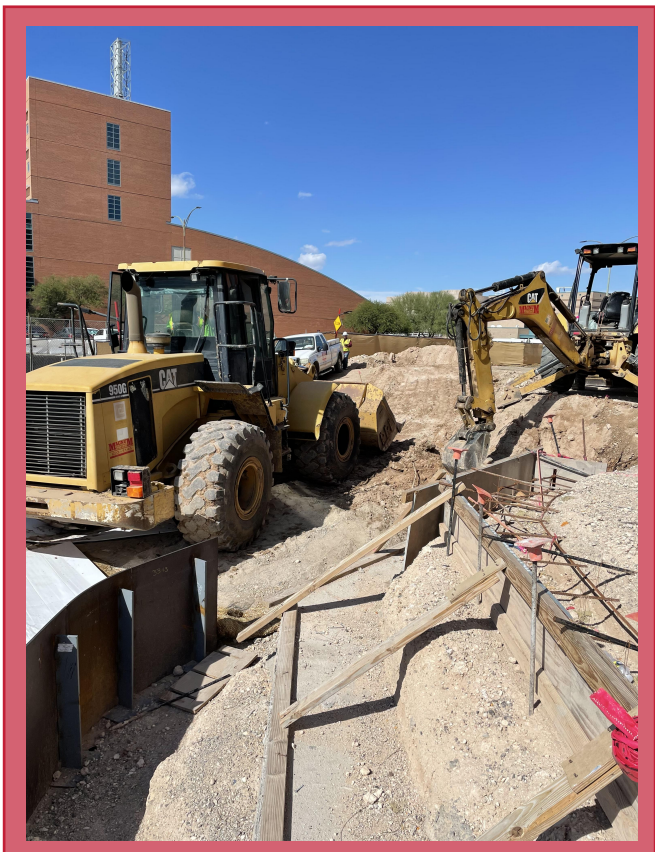
Using heavy equipment to achieve subgrade on West side
