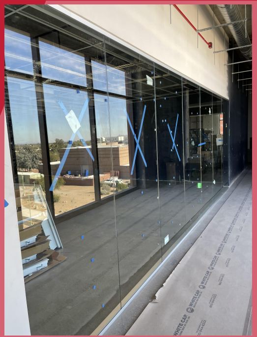
Interior Glass installed for clean rooms on Level 3
