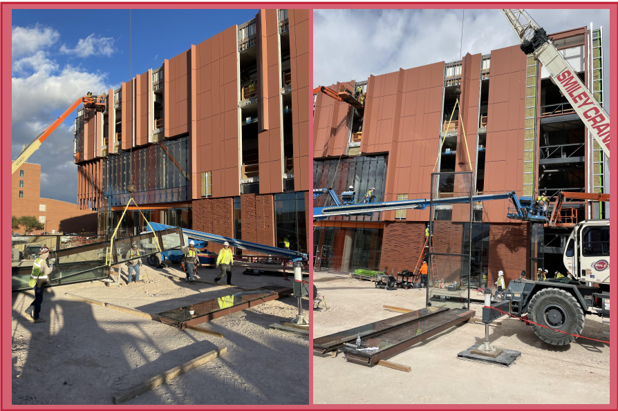
Flying panels of glass for the South elevation
