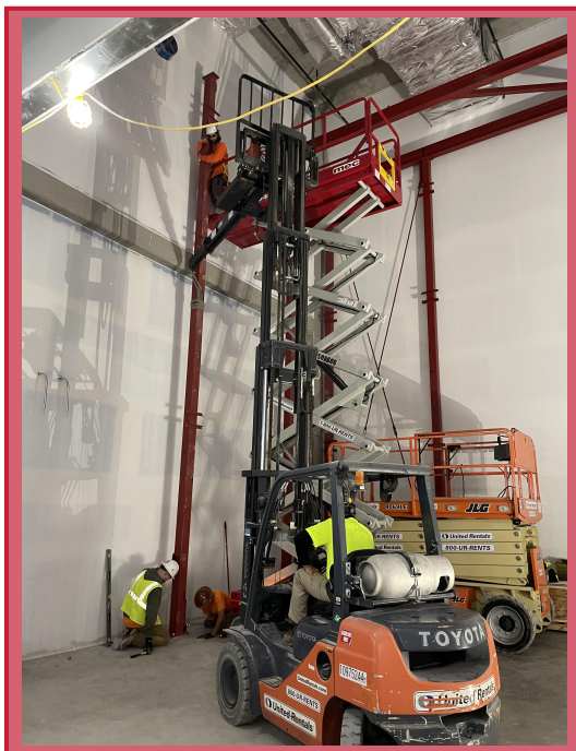
Using a warehouse forklift to erect steel columns
