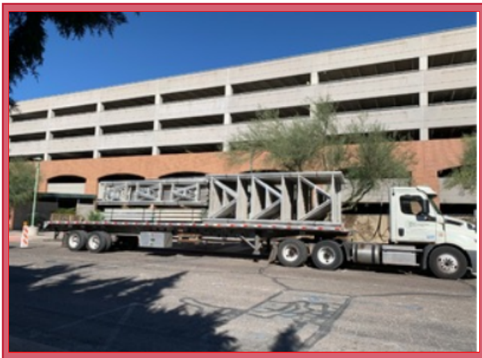
Additional Shoring Towers Delivered for Level 3
