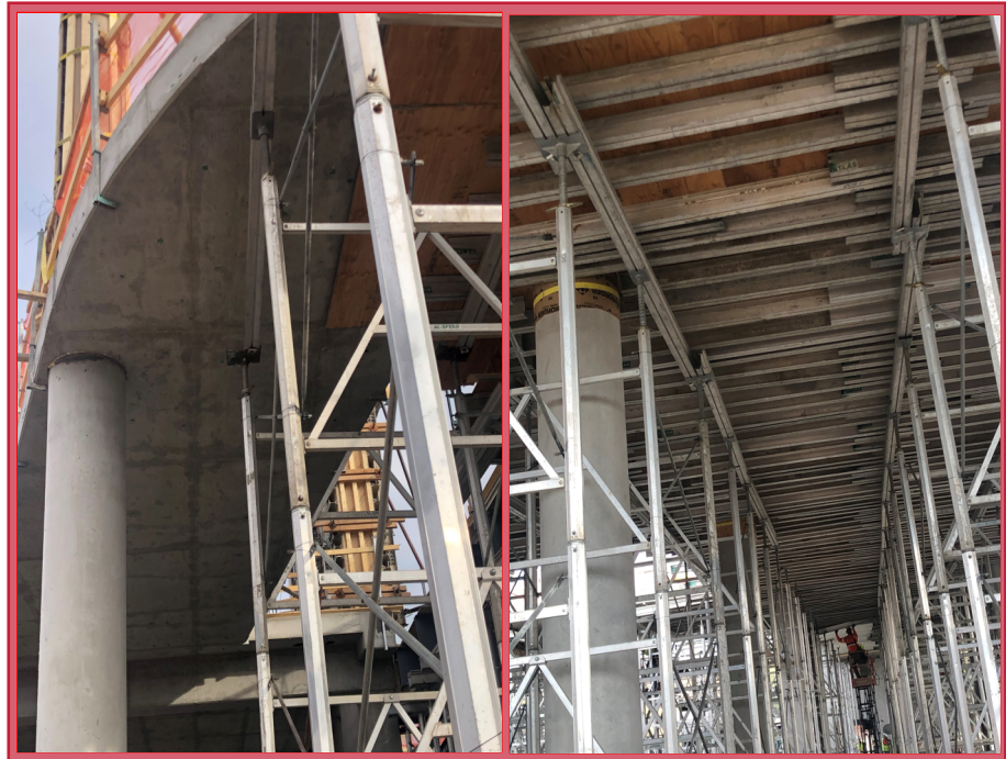
Level 2 Deck Stripping
