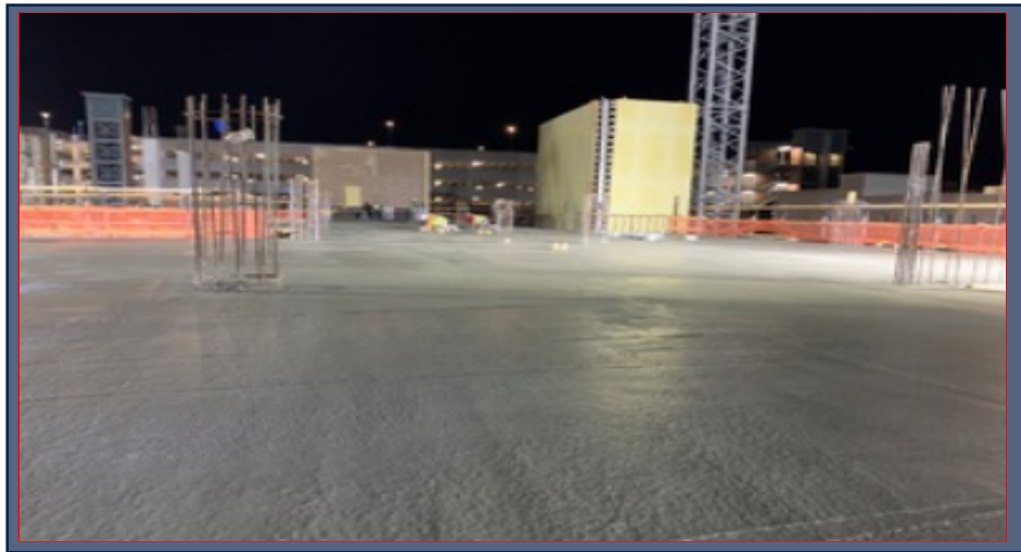
East Level 2 Deck is Poured
