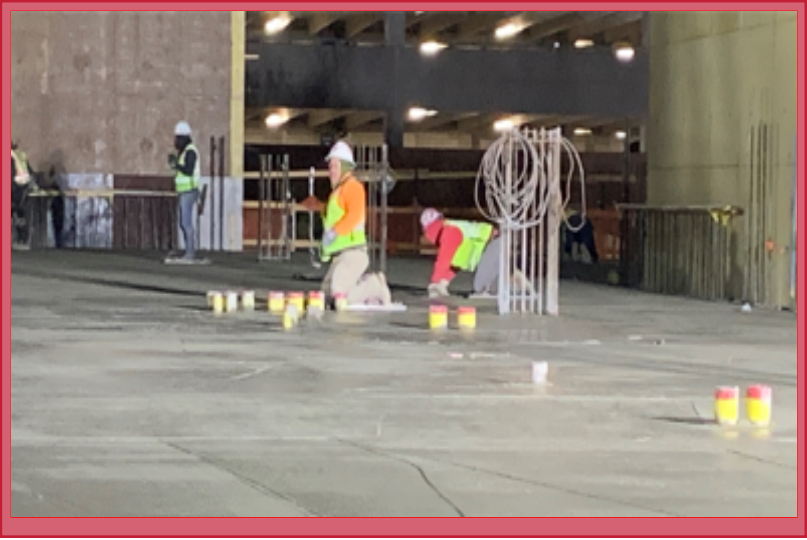
Mechanical/Plumbing Sleeves And Electrical In Columns
