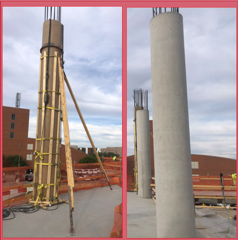
Forming and Pouring Level 2 Columns
