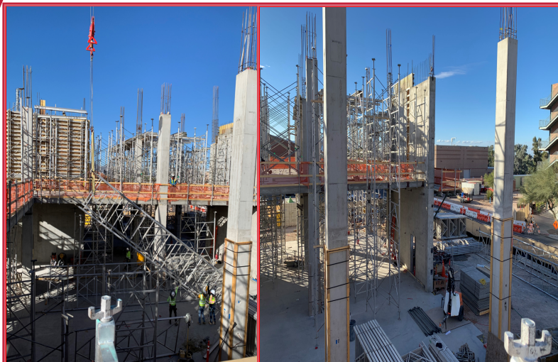
High-Bay (40') Shoring Towers Being Set
