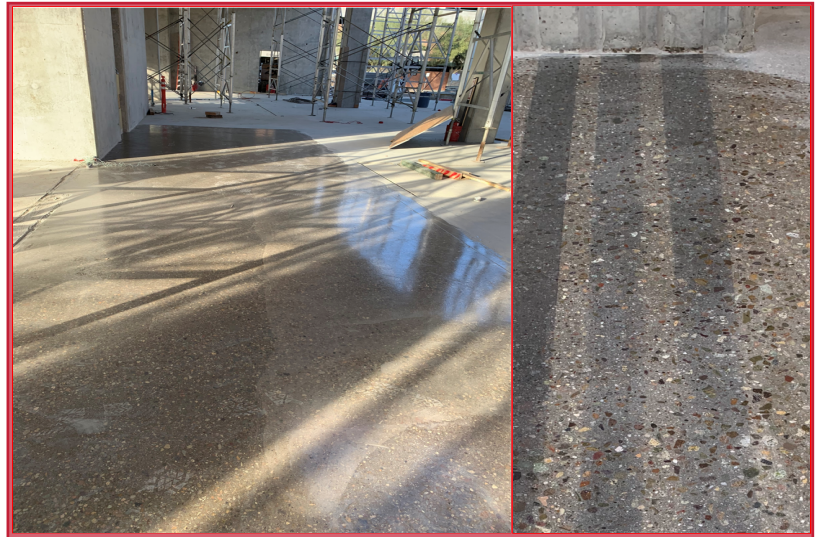
Level 1 Initial Grind and Mock-up of Stain Stripes
