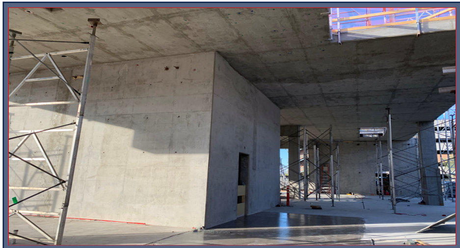
East Level 2 Deck Stripped
