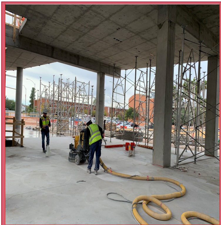
Forming and Pouring Level 2 Columns
