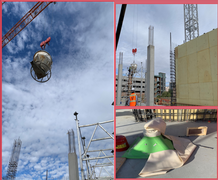
Pouring L2 Columns Using Concrete Bucket
