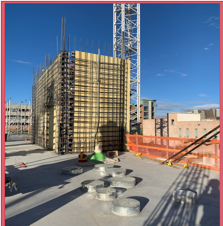
Mechanical Duct Risers Stub-ups
