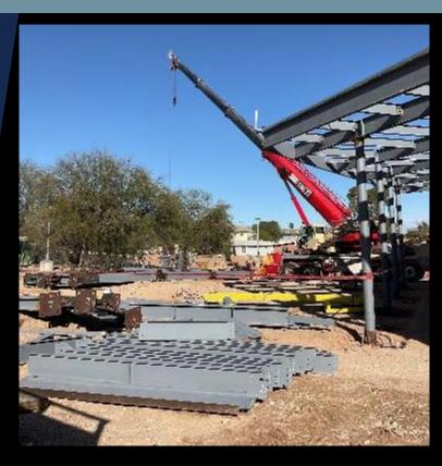
To aid in the steel erection on the office building a mobile crane has been brought to site and can be seen on the jobsite camera.
