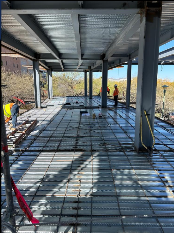
Office building Area A: Metal deck, rebar and concrete completed in level 2 & 3
