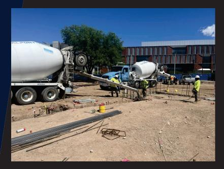
The entire concrete foundation for the Multi-Purpose building was placed in one day. Due to our wetter than normal monsoon season the Office Building foundation had to be broken up into 5 concrete placements.
