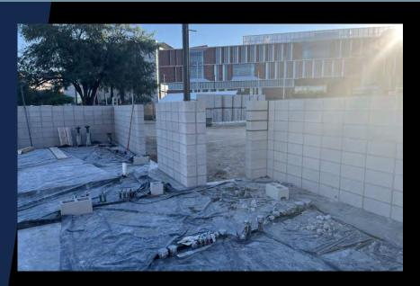
Now that the floor slabs have been placed, the masonry walls are being erected. The masonry walls will make up most of the structure in the multi-purpose and meditation buildings. On the other hand, the office building will have a steel structure, so the masonry walls are designed to absorb the shear(side to side) forces in the building.
