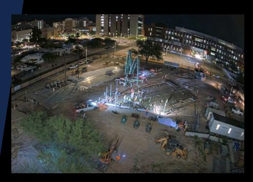
The concrete slab on grade was placed for all three buildings in two placements beginning at 3AM. During the hot summer months in Tucson, large concrete placements with significant surface areas are scheduled to begin early in the morning when the outside temperature is cooler. This ensures quality control and proper curing of the concrete.
