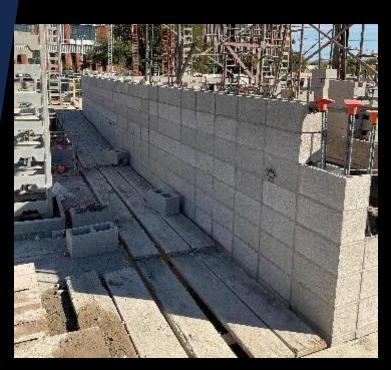
This month the CMU (Concrete Masonry Unit) walls are on their way up. These walls will be an exposed, finished product, so quality is critical. The architect and the UA Planning, Design, and Construction team are onsite regularly to perform inspections and help ensure that the quality is maintained throughout the entire process.
