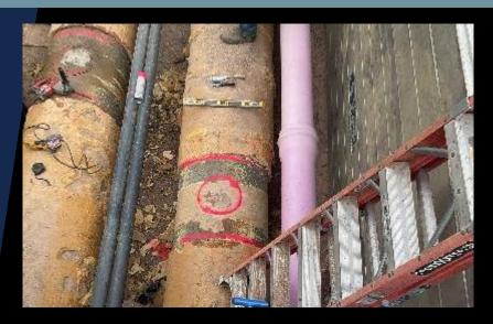
The University of Arizona campus has a network of different utilities, including chilled water lines that cool the air for Air Conditioning. This month we performed a "hot tap" on the main chilled water lines that run through the site for the connection that will feed AWCIM once complete. A hot tap requires coring into and connecting to an existing utility line while it is still in operation. Keep up with the project in real-time by looking at the live footage on the UA PDC website.
