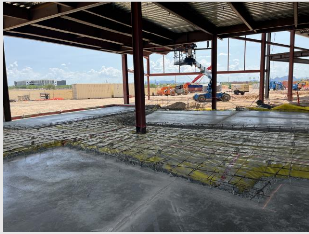
Depressed slab on grade placed
