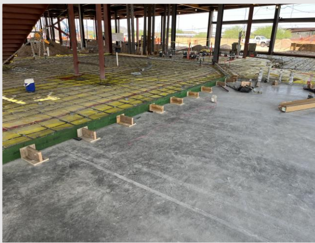
Upper slab on grade prepped
