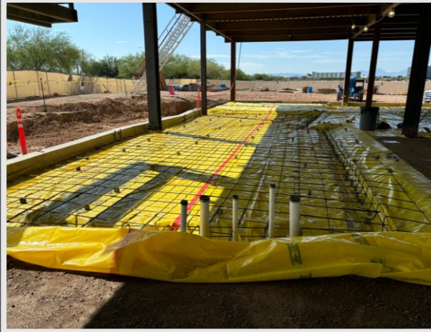
Depressed slab on grade prepped
