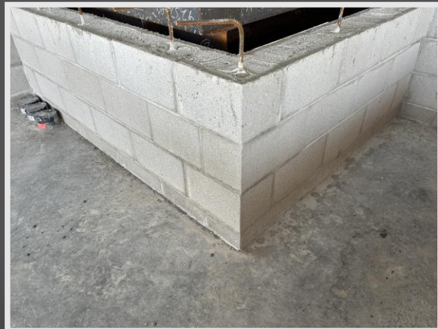
CMU block on the mezzanine of Studio A
