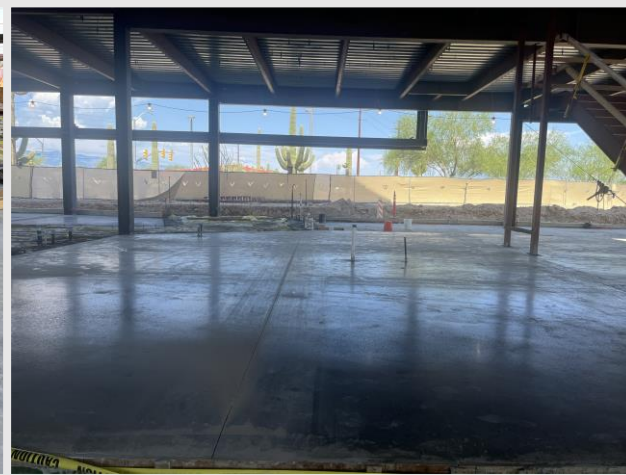
Upper slab on grade placed
