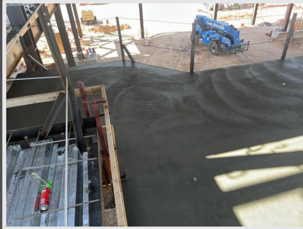
Slab on deck at mezzanine of Studio A
