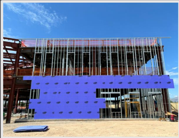
Start of sheathing
