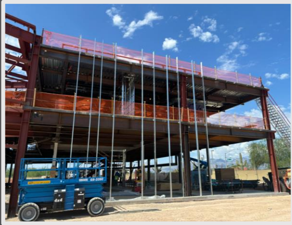
Start of exterior framing
