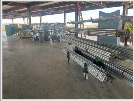
MEP Material Staging
