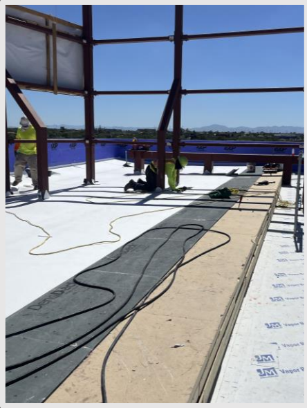
Foam slope build up
