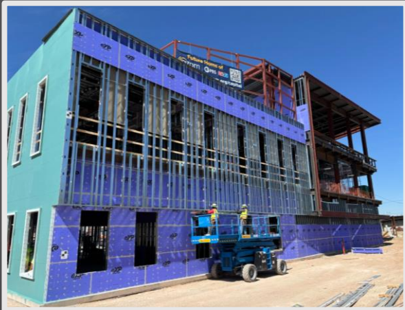
Exterior framing and sheathing
