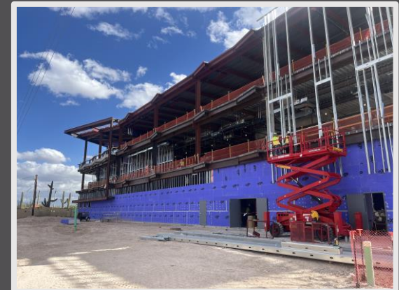
Framing and sheathing
