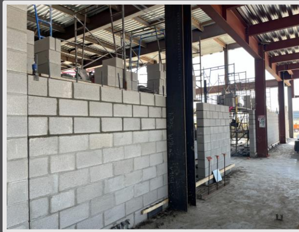
Beginning of CMU wall
