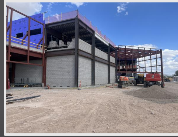
CMU in progress
