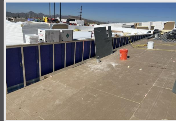
“Tippy-top” roofing in progress
