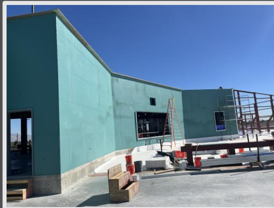
Vapor barrier over sheathing above
